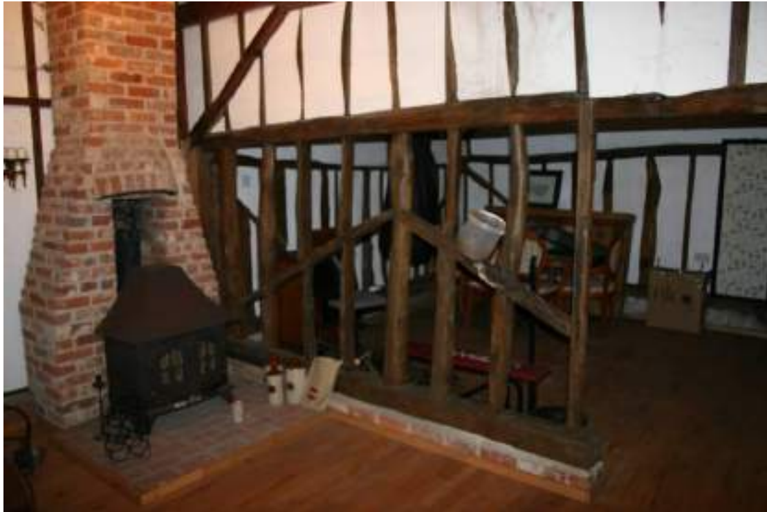
The timber-frame of the Forge. The studs have been truncated and raised on a plinth.
