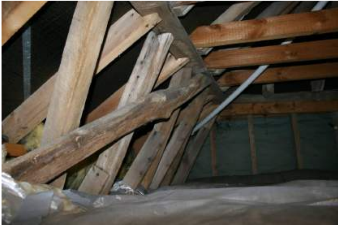
Some early timbers remain below the half pole purlin. Looking NE.
