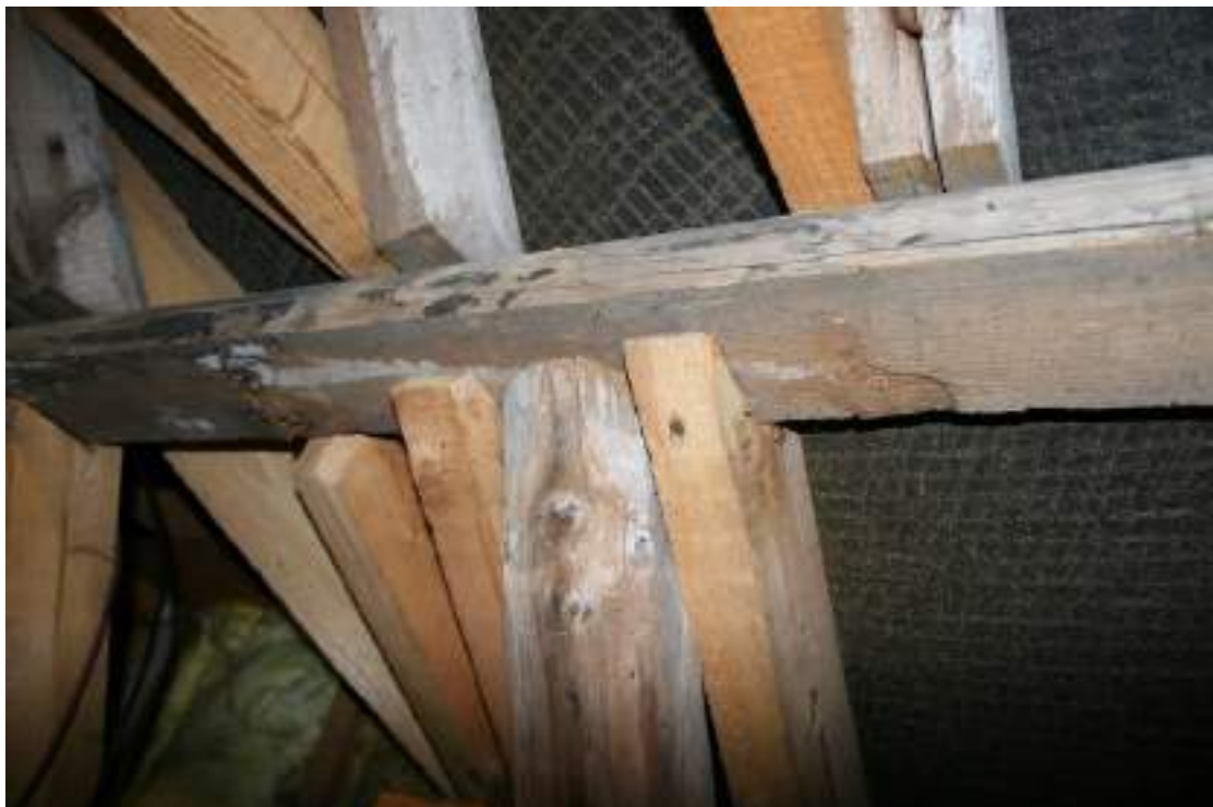
An early elm strut reused with later paired rafters above. Fresh timber dates to 1982.
