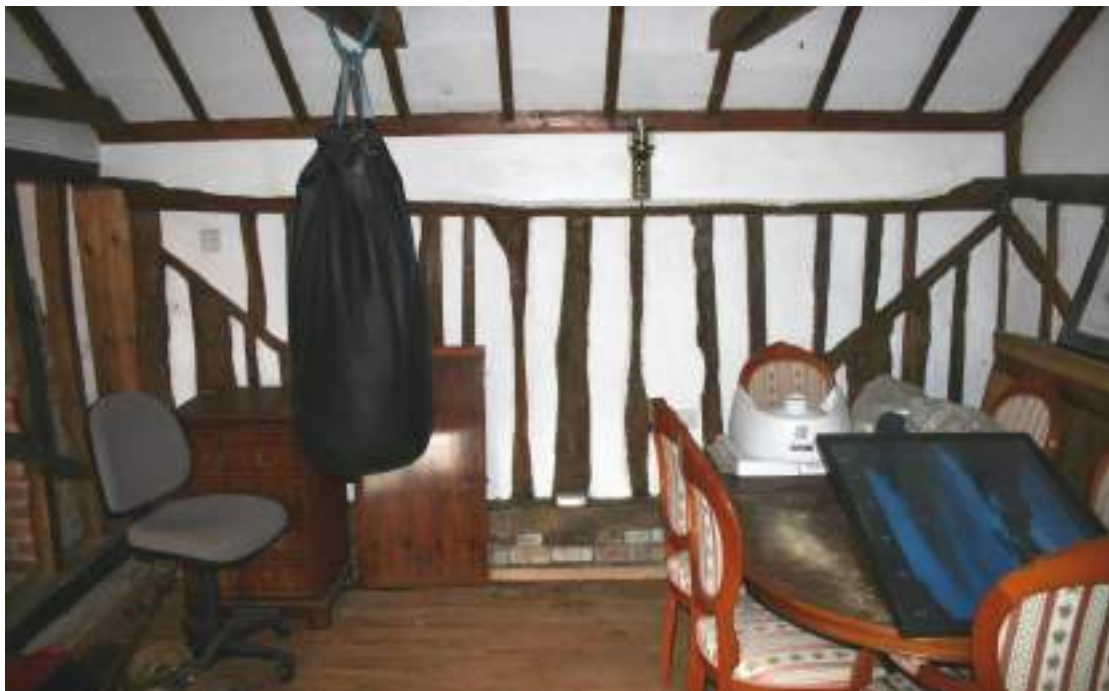
The NW wall of the Forge. Note the raised roof plate and modern roof.
