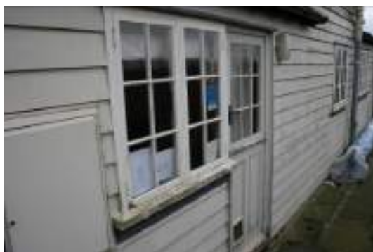
Detail of the rear windows and doors. Detail of the failing cladding.
