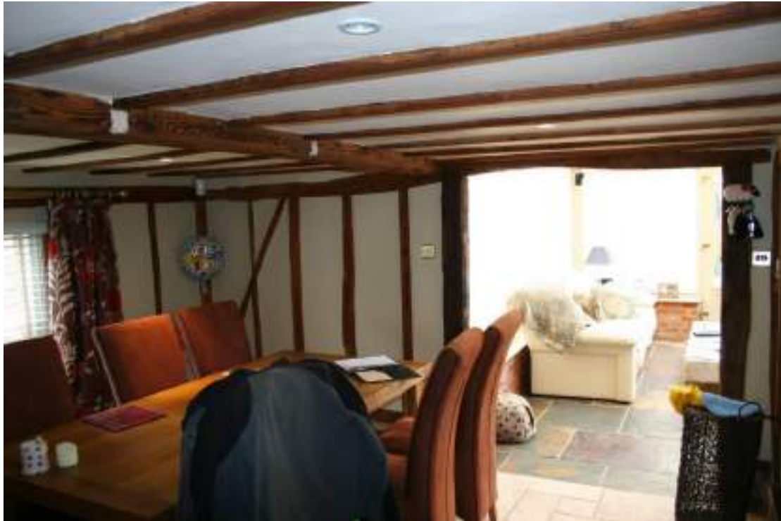
The Dining Room looking SW to the Garden Room. Note primary brace.
