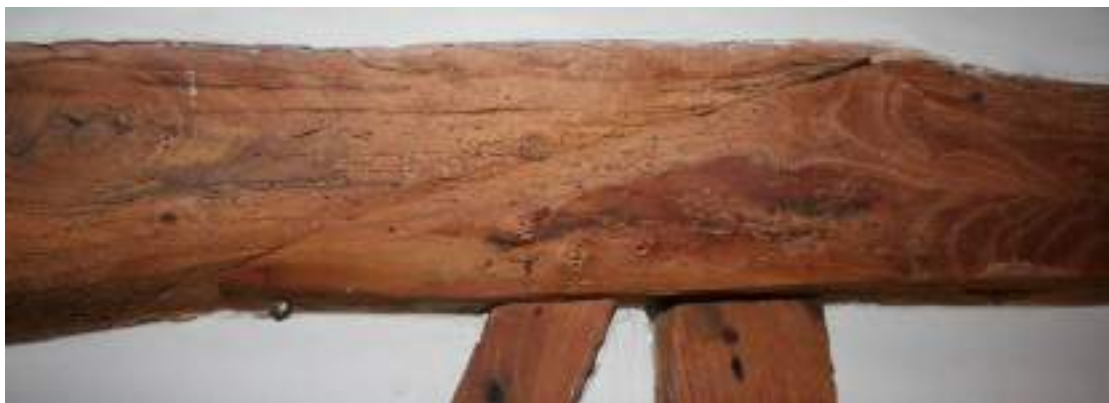
Clumsy scarf in the SW wall above the primary brace.
