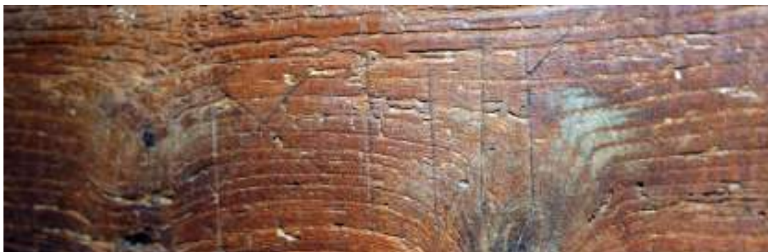
Carpenter's mark on the mid-rail visible in the Kitchen. Reads XIII(tag)
