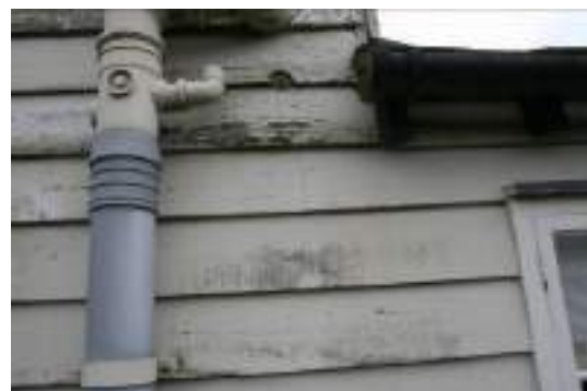
Detail of the rear windows and doors. Detail of the failing cladding.
