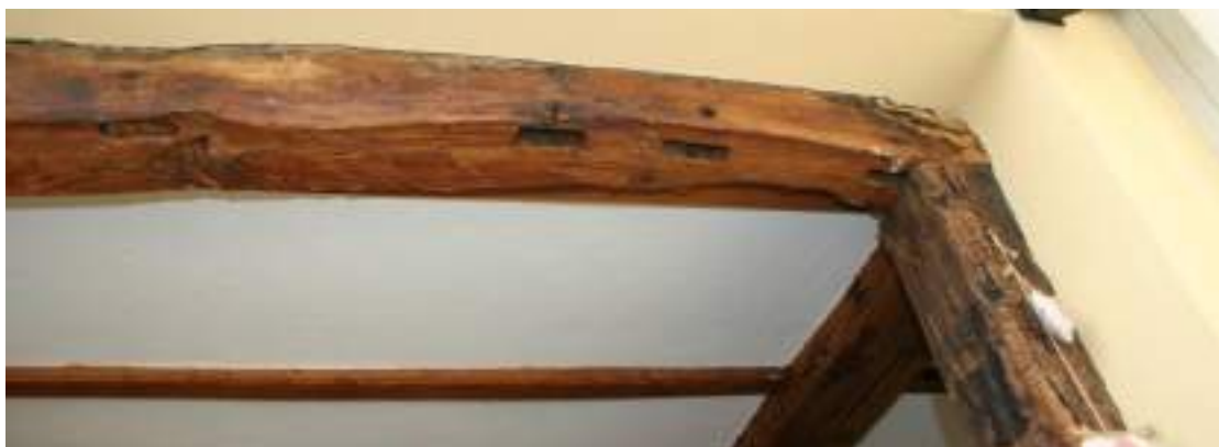
Looking upwards at the frame into the Dining Room. Note the rounded mortices.
