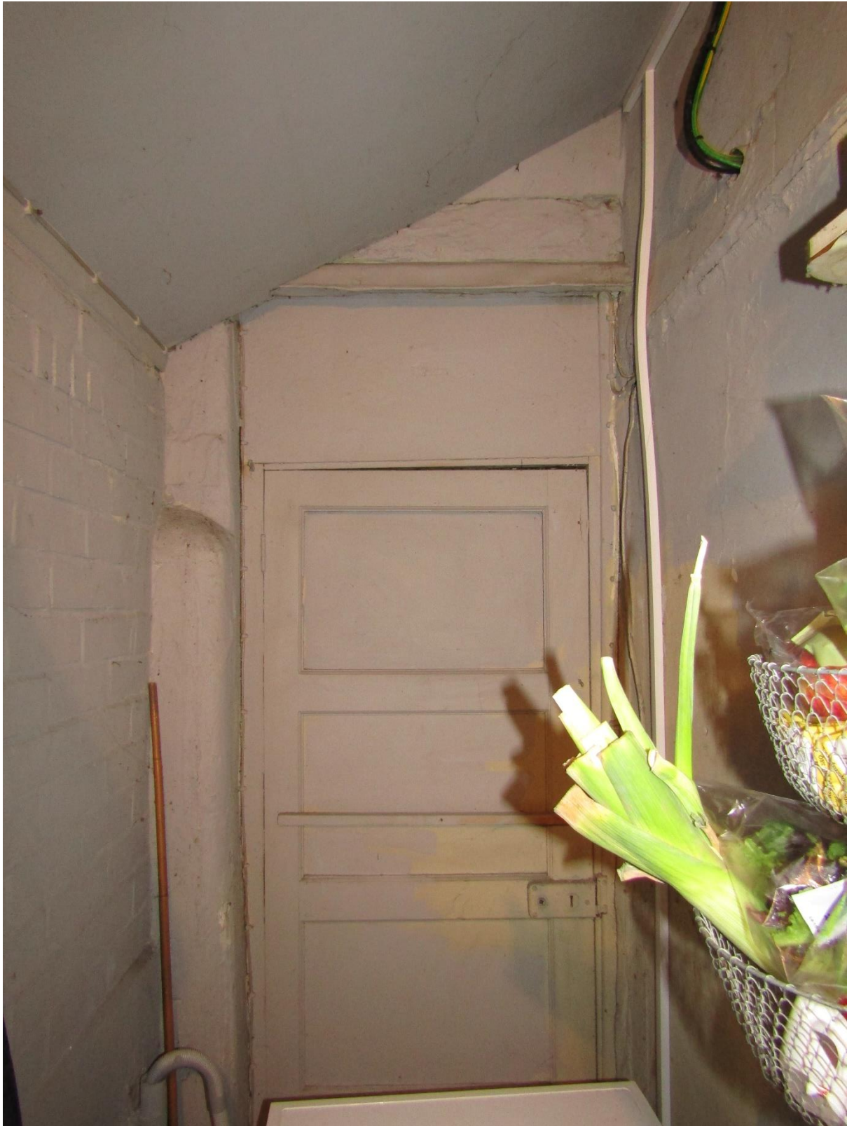
Figure 4 - infill section - door leading to property (now blocked off and forms cupboard)
