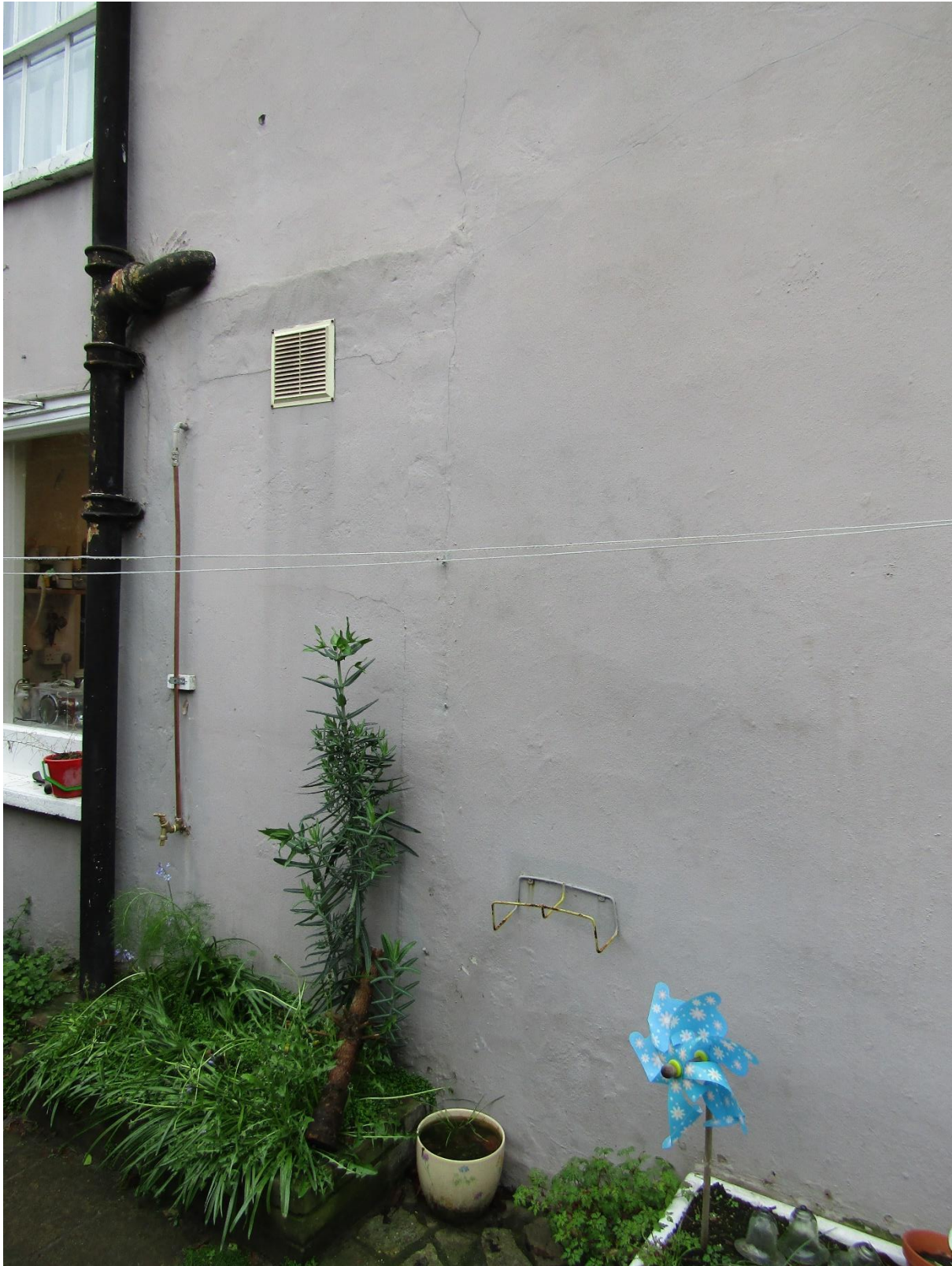
Figure 9 - rear elevation looking towards kitchen window. Evidence of a former opening in render
