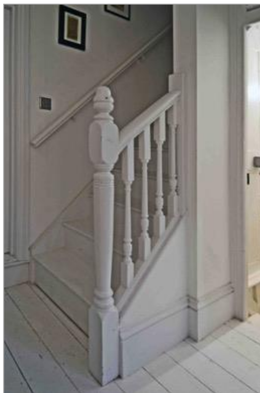
Fig. 4 Newel post and balusters Joinery to a typical late 19 th – early 20 th century pattern
