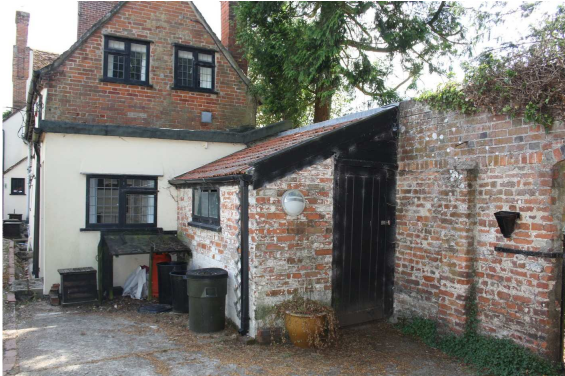
The north end. The ground floor window to be replaced with an external door, the First Floor windows are to be replaced. The shed is to be clad in vertical boards, the window replaced and the shed door is to become a window.
