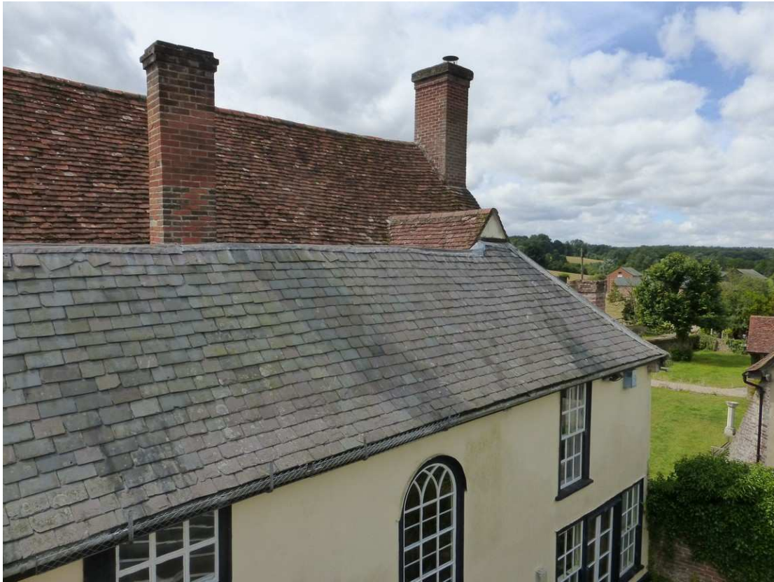
The slate roof and lead ridge are in a very poor condition at the north roof pitch
