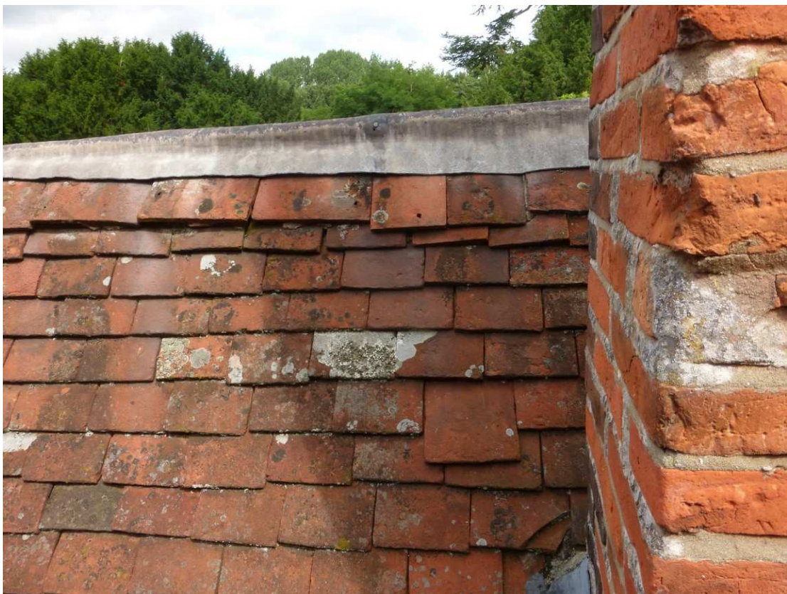
The slate roof and lead ridge are in a very poor condition at the north roof pitch
