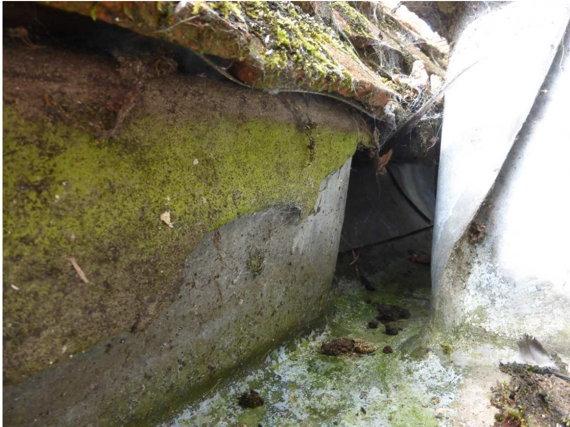
Detail of the outflow point of the rainwater chute into internal valley gutter, behind the chimney
