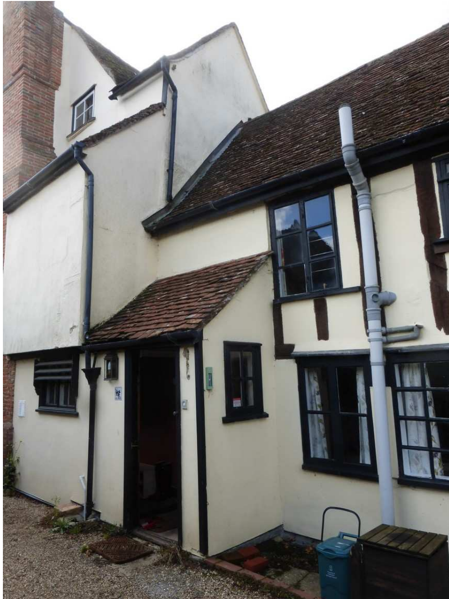
View of the side door arrangement. The soil and vent pipe and wastes are to be removed.
