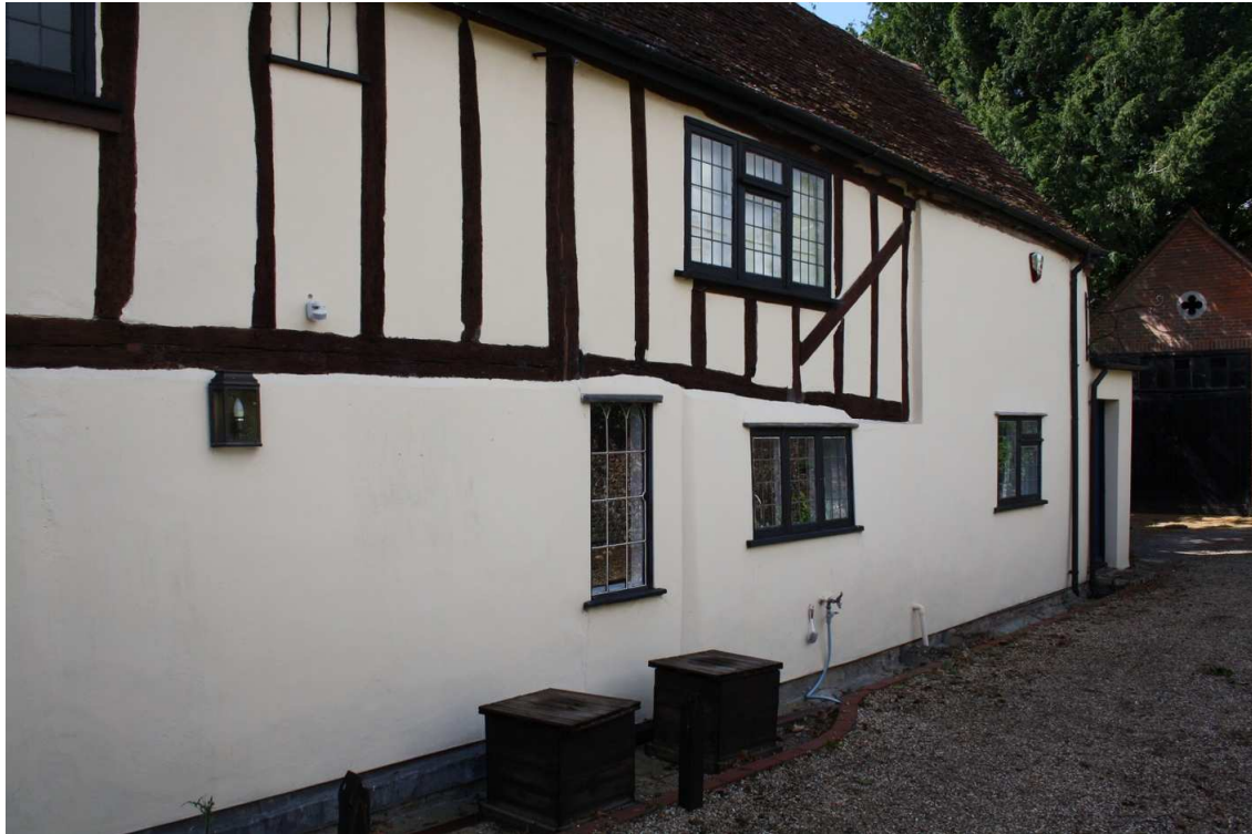
The east side showing windows for replacement. The gothic headed iron window is to remain.
