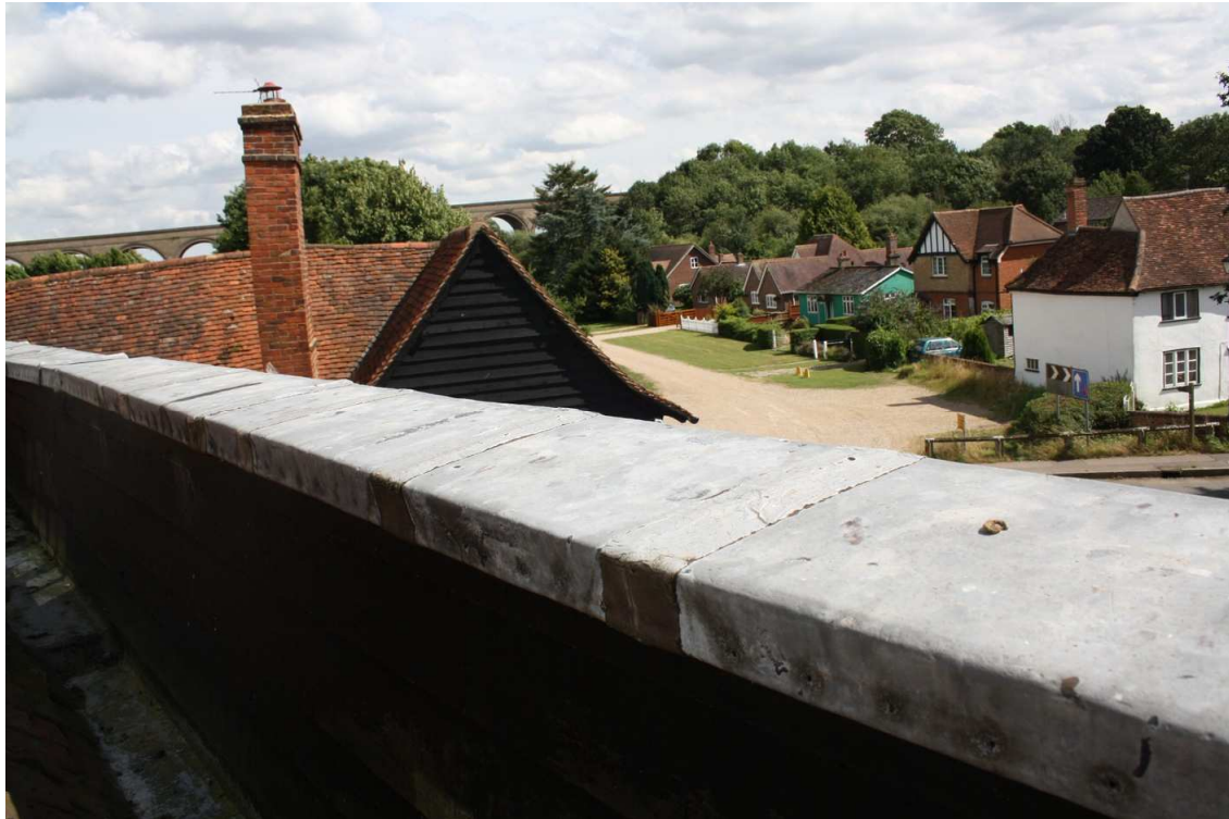
Replacement of the south parapet coping. The coping is heavily repaired with flashband.
