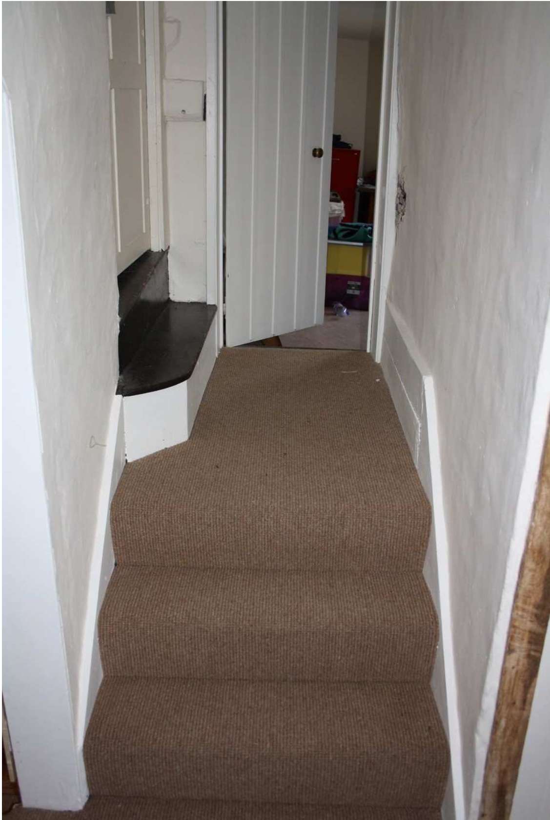
The up and over platform at the attic stair. The whole platform is to be removed and a new opening formed in the wall at the right of this view. The attic stair is to have new winders and the door to the new Library (straight ahead) is to be replaced.
