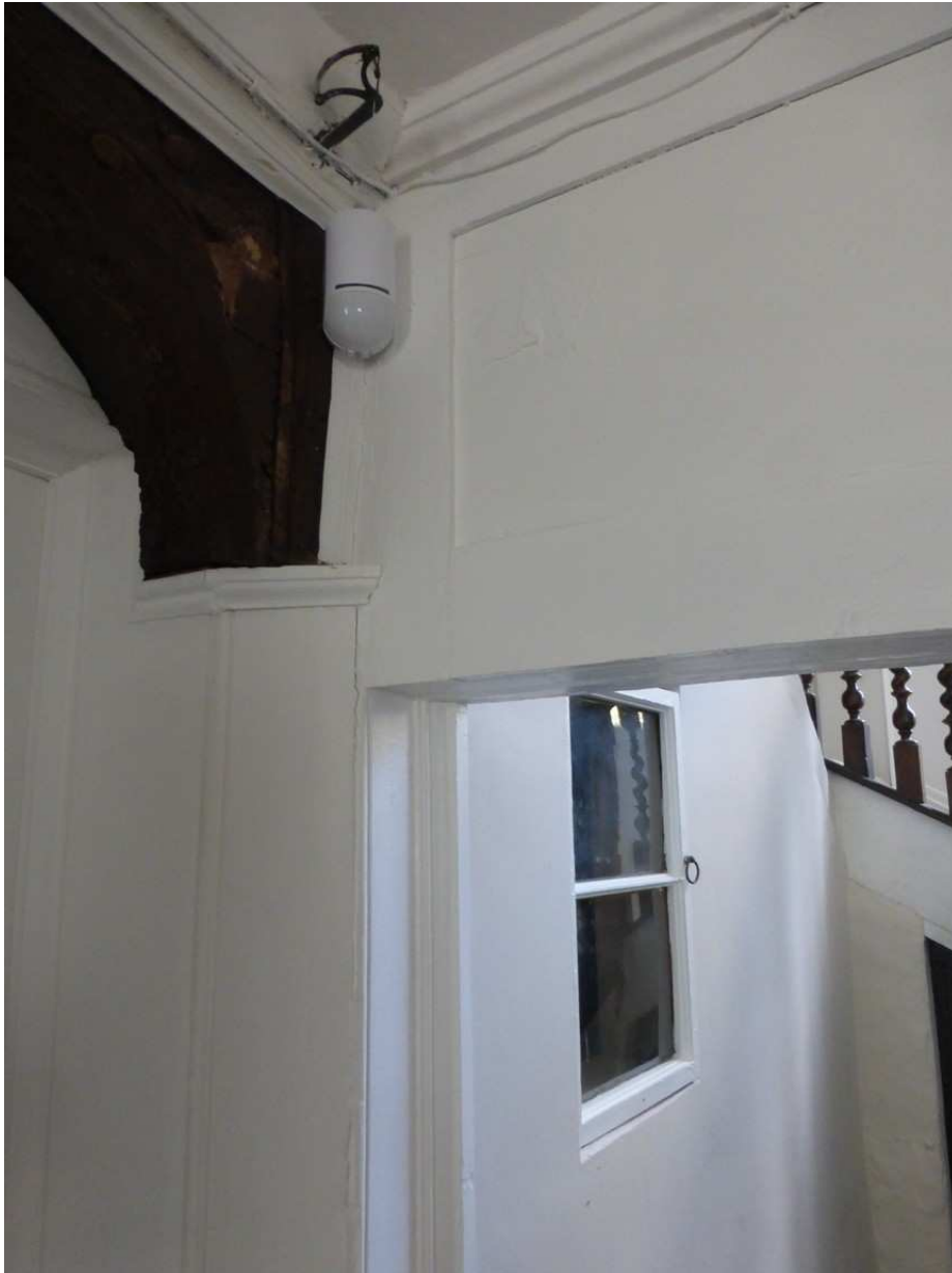
Improvement of mouldings in the Hall - the arch over the door to the Drawing Room. A variety of off-the-shelf mouldings have been used as make-shift repairs and it is intended to replace the worst offenders.
