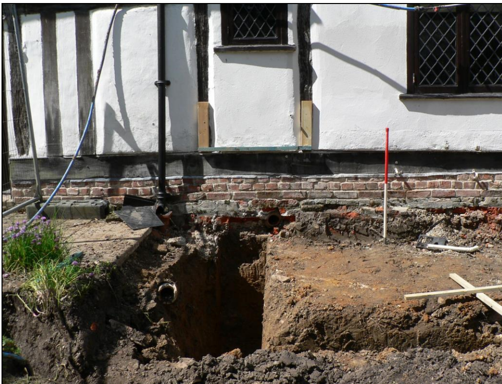
Southern side of trench foundations on NE side of building with c1900 brick foundation below replacement timber plate
