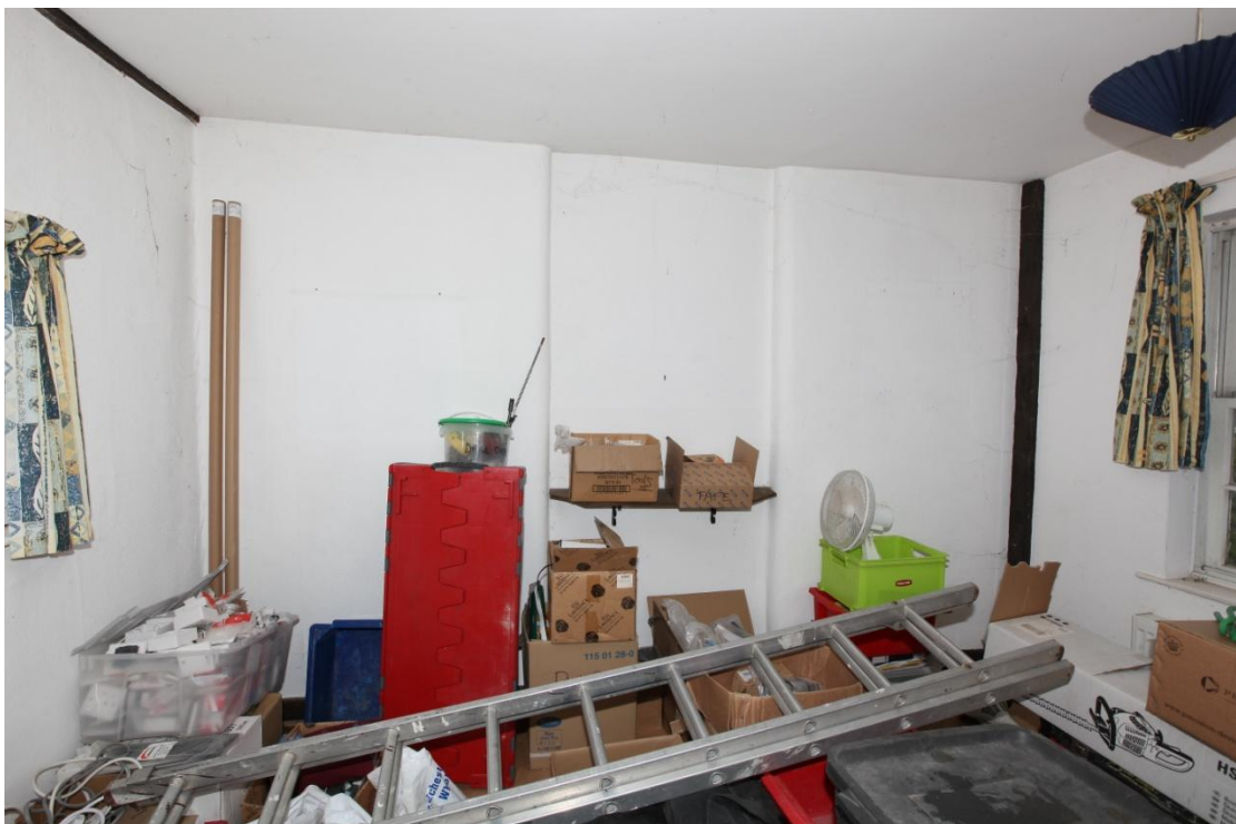
Illus. 14. The western internal gable of the western bedroom (2f) showing the unusual central recess indicating the position of the chimney. A fireplace may have been removed from this position. The timber to the right is a 20 th century Mock Gothic insertion.
