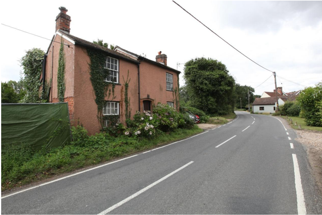
Illus. 3. The house from the north-east showing the uniform peg-tiled roofs of the building's two sections with shallow pitches more usually intended for slate. The gable chimney of the taller western section is wide enough for two flues but its counterpart on the east only one.
