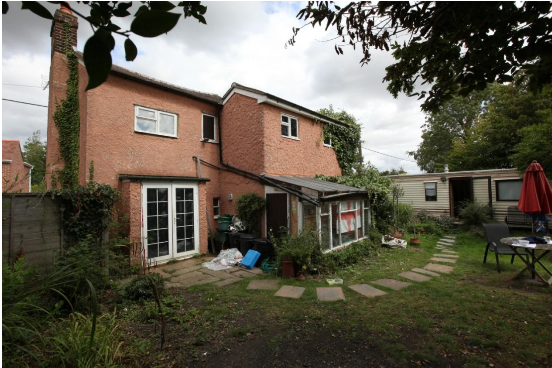
Illus. 5. The building from the south-west showing its late-20th century windows, French doors and conservatory with the narrow pitched roof of the mid-20th century rear extension (3) in the centre.
