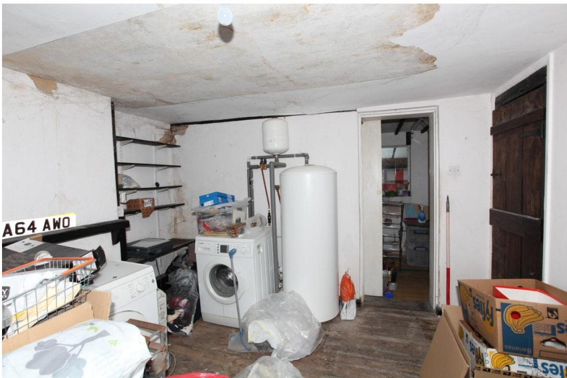
Illus. 8. The dining room (1) from the north showing the door to the kitchen (3) in the centre with an under-stair cupboard on the right and the gable fireplace on the left. The fireplace is blocked and lies beneath a 20 th century Mock Gothic wooden shelf. The narrow pine floorboards are identical to those of the lounge (2) but the height of the dining room floor is 10 cm lower (4 ins).
