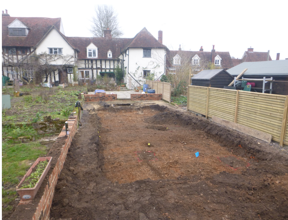
Photograph 1 Site shot, fully-excavated, looking east
