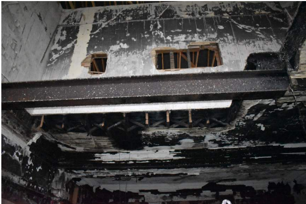
Plate 25 Metal beam that would have supported the floor of room 22 prior to the fire. Herringbone strutting visible behind - view south-east.
