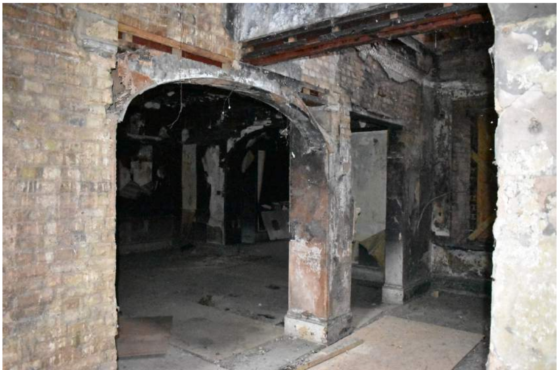
Plate 26 Inserted arch leading into bar with removed wall to right, both supported by metal beams - view west.
