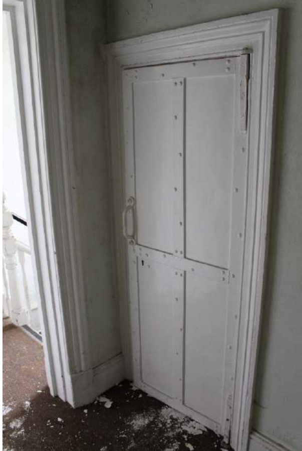
Plate 17 Iron door to strongroom 20, converted from the former servants' quarters for Officers Nos.2 and 3 - view west. Photo from November 2013 left, photo from December 2019 right.
