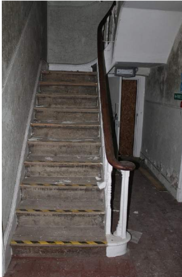
Plate 21 Stairwell v, the basement stairs with the same mahogany banister with spiral end and turned balusters as the staircases of the entrance ways – view north-west. Photo from November 2013 left, photo from December 2019 right.
