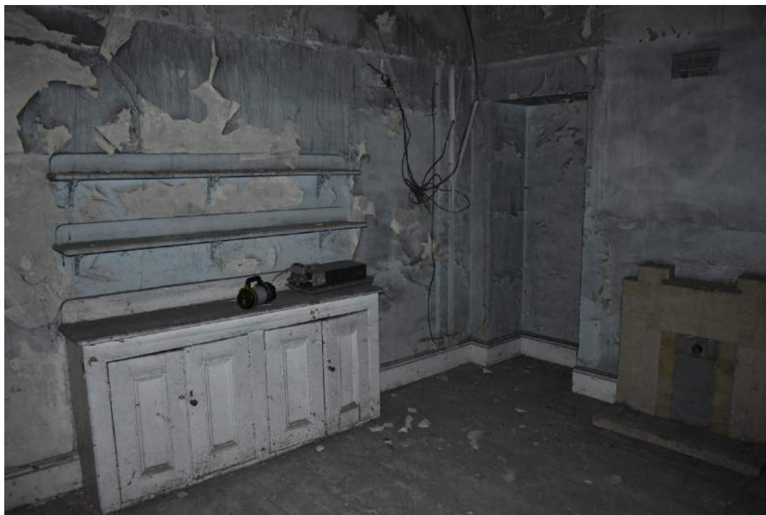
Plate 16 Room 18, formerly quarters for the servants of Officers Nos.1, 6 and 7, showing the bricked-in original doorway to the left of the chimney breast and the double-width dresser on the dividing wall – view south. Photo from November 2013 above, photo from December 2019 below.
