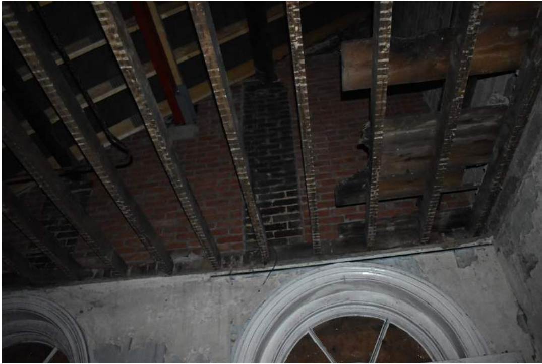
Plate 29 Engineering brick columns supporting purlins socketed into gable brickwork above room 19 - view south-east.
