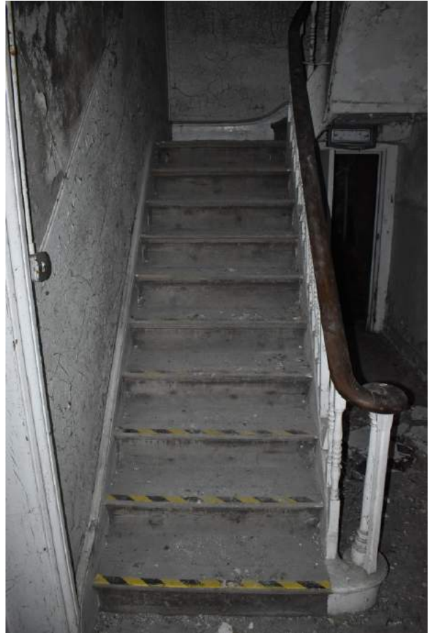
Plate 21 Stairwell v, the basement stairs with the same mahogany banister with spiral end and turned balusters as the staircases of the entrance ways – view north-west. Photo from November 2013 left, photo from December 2019 right.
