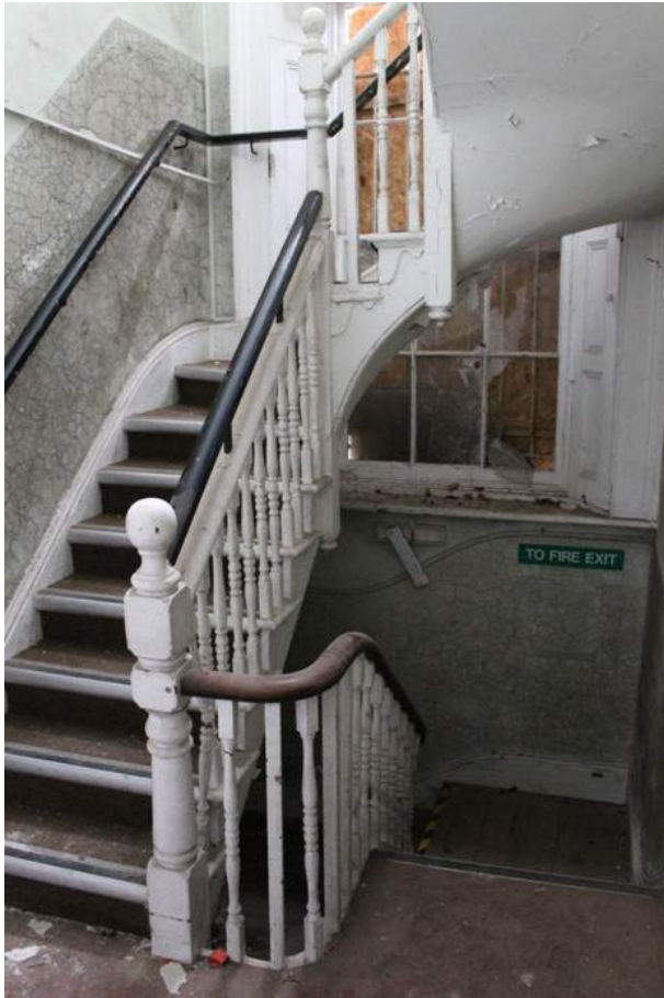
Plate 11 Servants' stairwell v, with the original access to the basement and the inserted staircase to the first floor - view west. Photo from November 2013 left, photo from December 2019 right.
