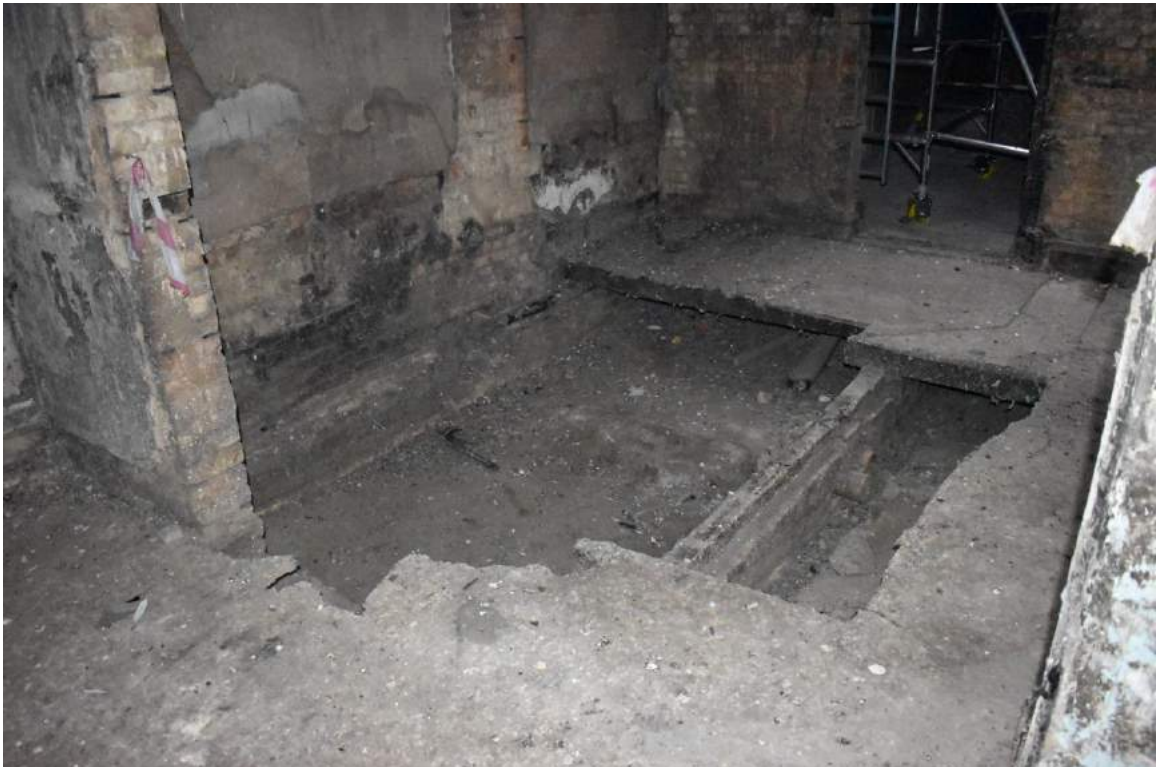
Plate 24 Missing floor in ground-floor on building below room 24, with exposed brick plinths - view north.
