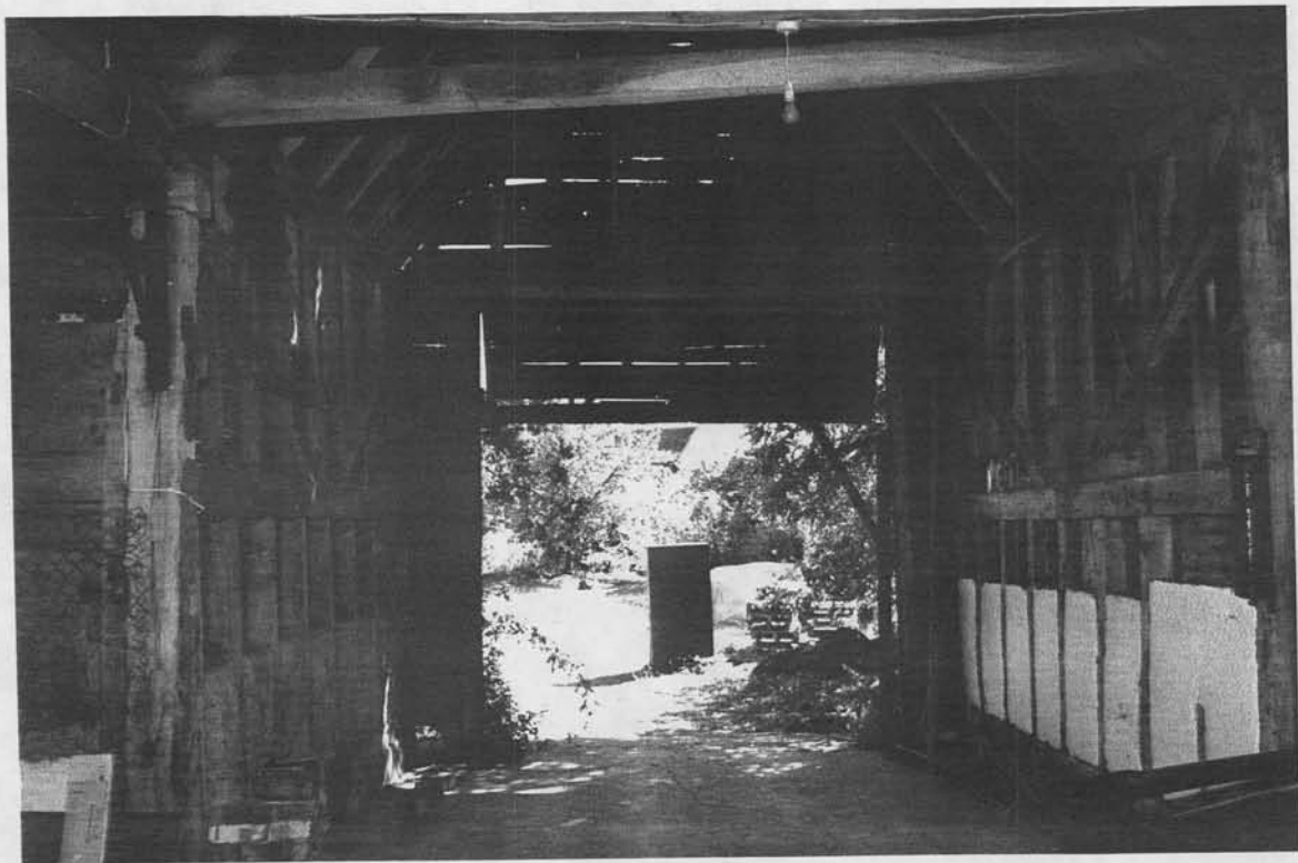
Plate 15 Truss 6: view showing mortice for angle tie on tie beam, also showing adjoining piece of top plate (replacement as there is no joint for angle tie on top face).
