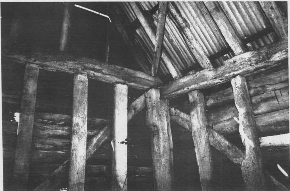
Plate 14 Truss 1: view showing joints for angle tie
