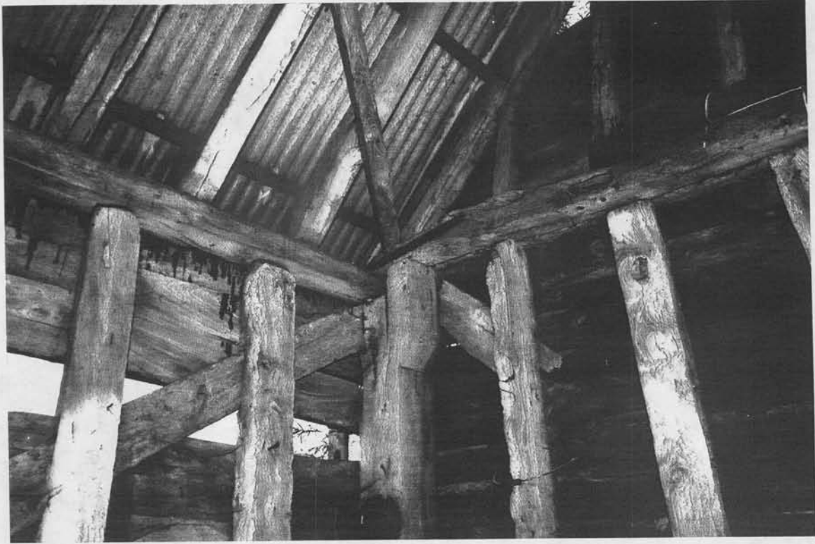
Plate 15 Truss 6: view showing mortice for angle tie on tie beam, also showing adjoining piece of top plate (replacement as there is no joint for angle tie on top face).
