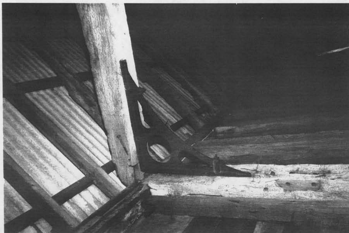
Plate 11 Truss 2: detail of knee and jowl
