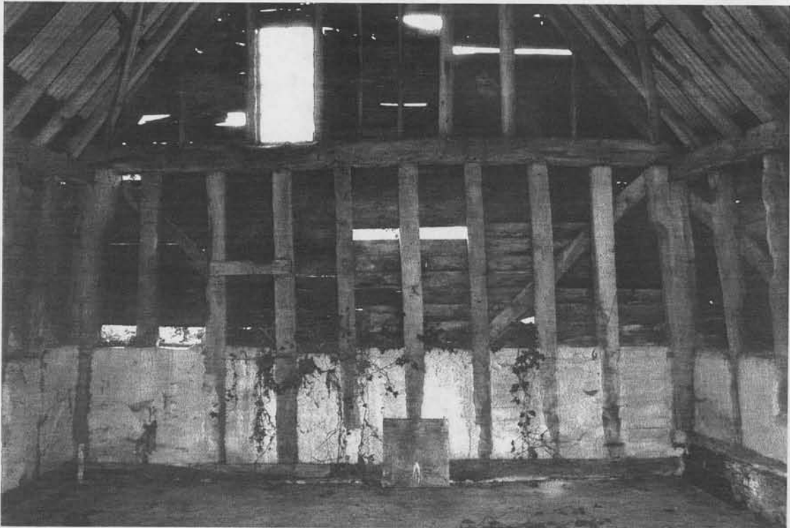
Plate 8 Truss 1 (end truss)
