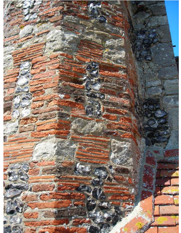
Fig. 5 Detail of the staircase tower, rebuilt after the 1884 earthquake. Although modern brick has been left exposed in the interior, the exterior uses tile and narrow brick as seen elsewhere on the tower.
