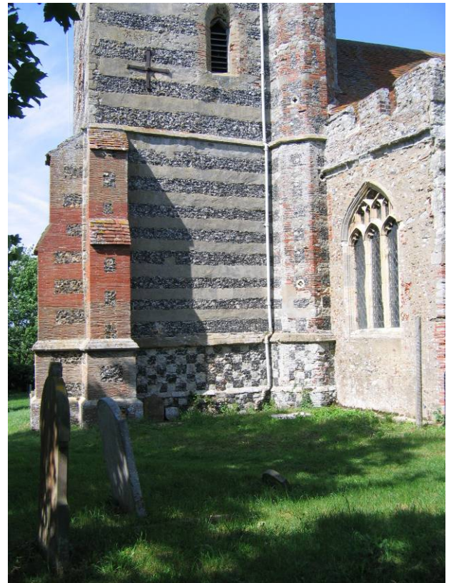
Fig. 2 The two buttresses built under the supervision on Wykeham Chancellor in 1920. They have since been repaired with modern tiles.
