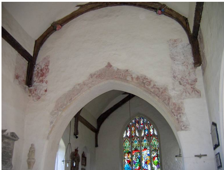
Fig. 3 The chancel arch with wall paintings uncovered following the 1884 earthquake and the unusual timber roof with carved portrait heads on the spur ends.
