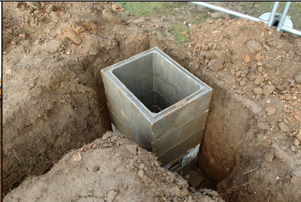
Catch Pit 3 / settling tank
