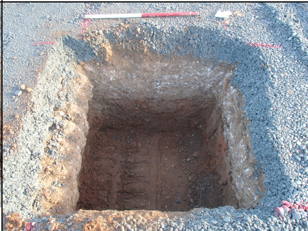
Construction pit for Floodlight Base 3
