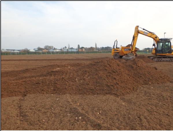
Topsoil stripping in progress
