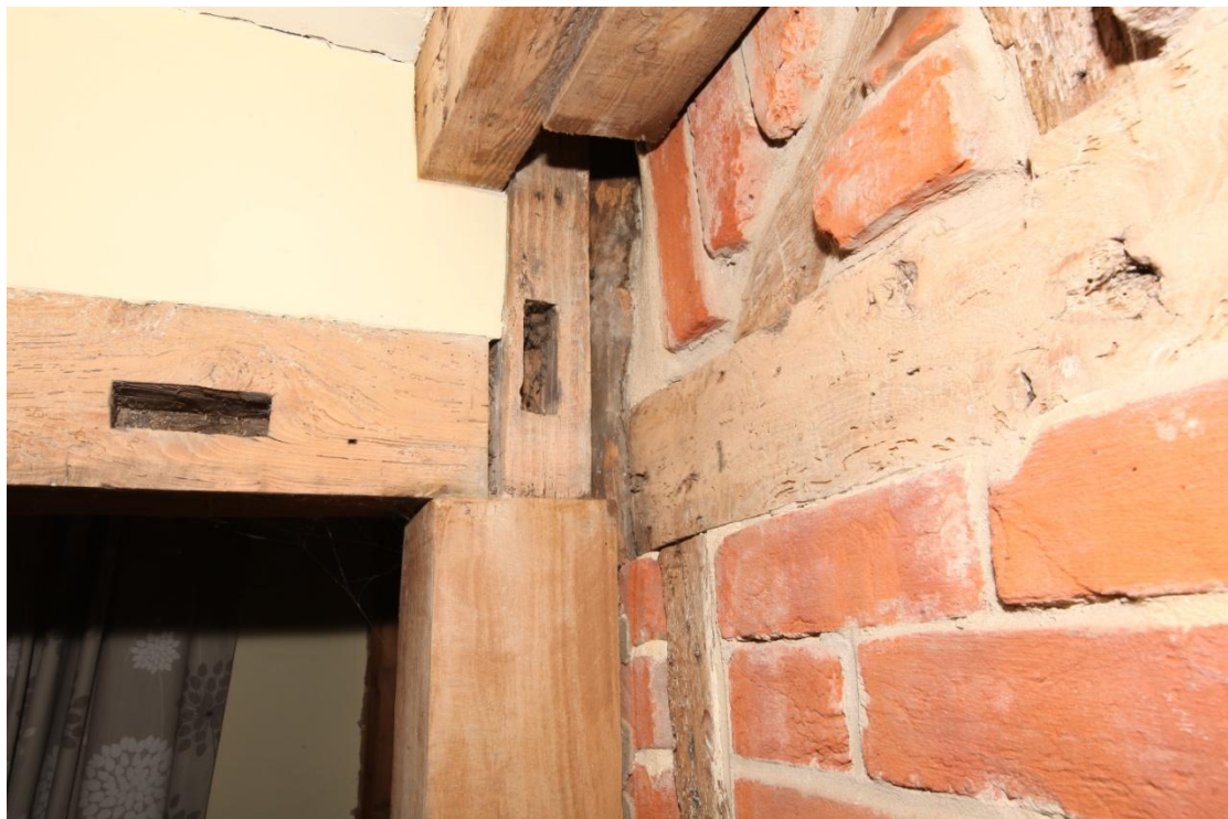
Illus. 8. A detail of the left-hand post in illus. 7 above, showing the original south-western corner post of phase 1 hidden behind it. The pegged joint between the post and the gable mid-rail is visible in the centre of this image, but the diagonal primary brace is nailed rather than pegged in the typical manner of the early- to mid-19 th century.
