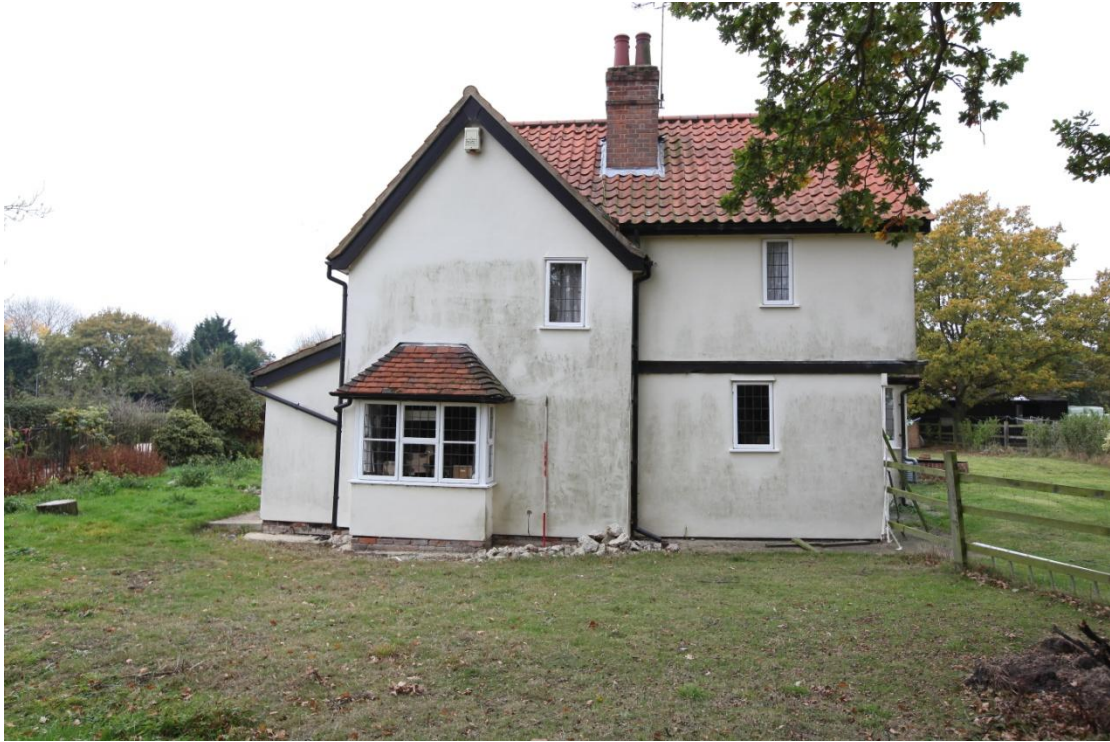
Illus. 3. The building from the east with the original 19th century gabled structure to the left (1) and the north-eastern rear extension (2) on the right.
