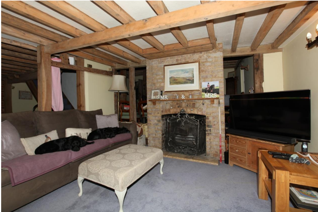
Illus. 9. The rear (northern) interior of phase 1's eastern bay (1b) showing the gault-brick arched fireplace and chimney of phase 2. The chimney is respected by the present ceiling, which replaced the original ceiling at the same time.
