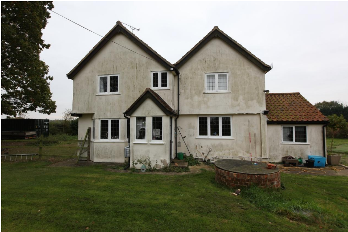
Illus. 4. The rear (northern) elevation showing the two gabled rear extensions (2 and 3) after the removal of the Mock Gothic false timbers shown in 1983 (figure 11). The central rear porch and the single-storied kitchen extension on the right (3a) were built after 1983.
