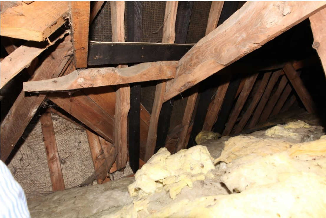
Illus. 16. The original clasped-purlin phase 1 roof structure with a nailed collar at its hipped western end, as seen from the south. The pine timbers, both stained and unstained, are modern additions. The 20 th century softwood and cement render of the north-western extension (3) is visible at bottom left.
