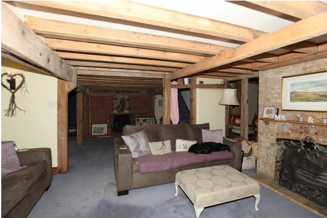
Illus. 5. The interior of the original two-bay building (1) looking west from its eastern gable. The ceiling and the chimney of the eastern bay on the right date only from the addition of the rear wing (2) after 1923. Some of the timbers at the foot of the staircase may survive from the original central partition but the southern wall to the left has been entirely removed where it adjoins the later lean-to extension (4).
