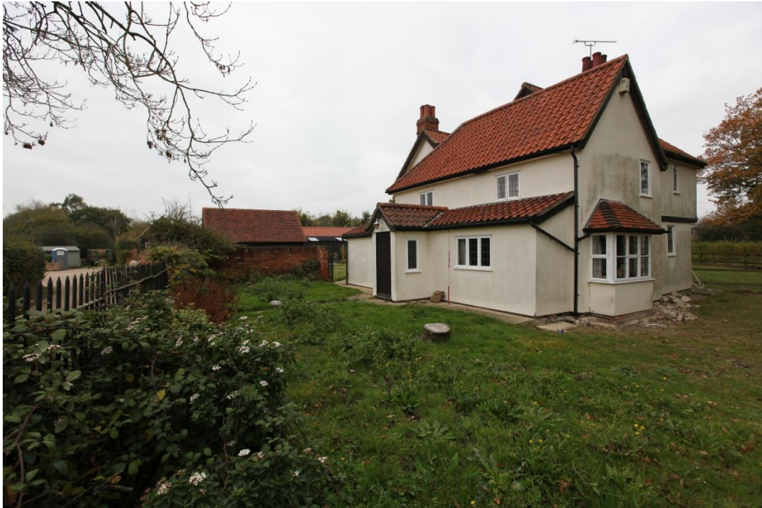
Illus. 1. Heathwell House from the south-east showing Stone Lane on the left. The building's uniform appearance is the product of an extensive late-20 th century or early-21 st century restoration which disguised its complex origins with new windows, pantiles and cement render.
