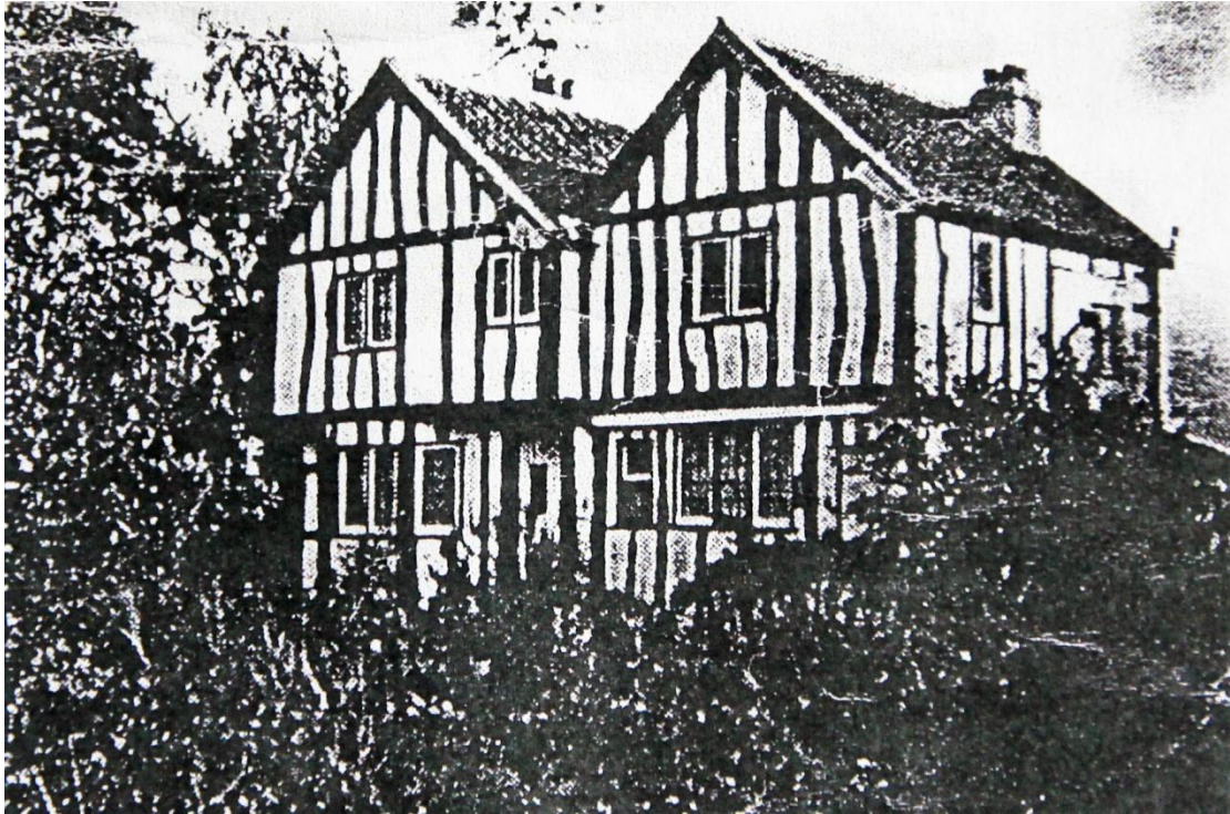
Figure 10c. The rear (northern) elevation in 1983, showing the false timbers to both the eastern and western rear wings (2 and 3 respectively). The rear porch had yet to be added, and the waney, misshapen timbers are typical of the Mock Tudor fashion of the 1920s and 30s. The irregular shape of the two extensions, with the left-hand wing projecting slightly further than its neighbour, suggests they were built at slightly different dates and possibly when the property was still divided into tenements. Each wing replaced the probably original lean-to sheds that were still present in 1923.
