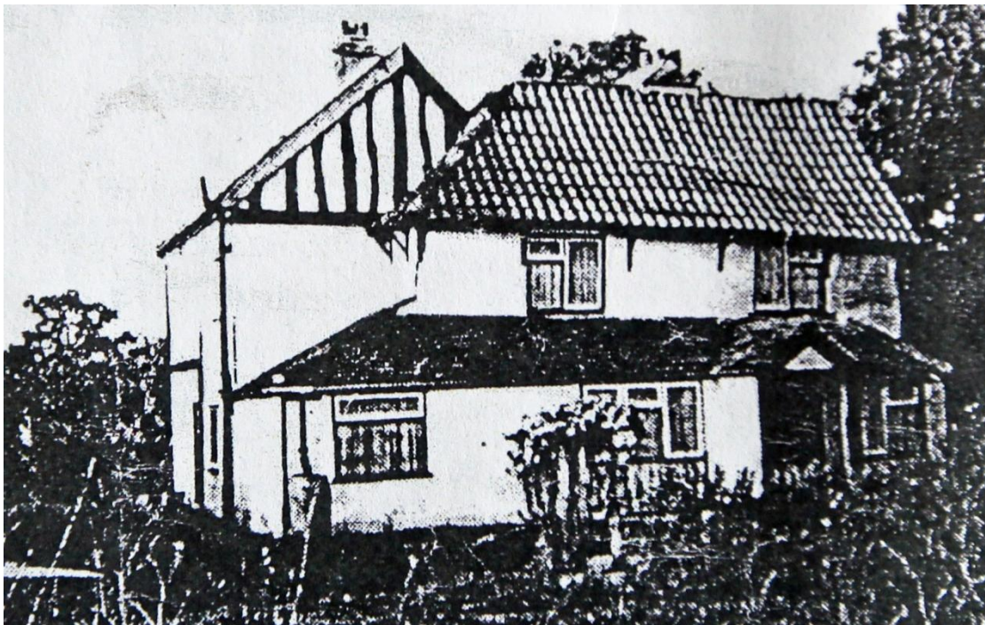
Figure 10b. The house from the south-west in the 1983 particulars, showing the false timbers to the gable of the western rear extension (3). The western kitchen extension (3a) had not been added at this date.
