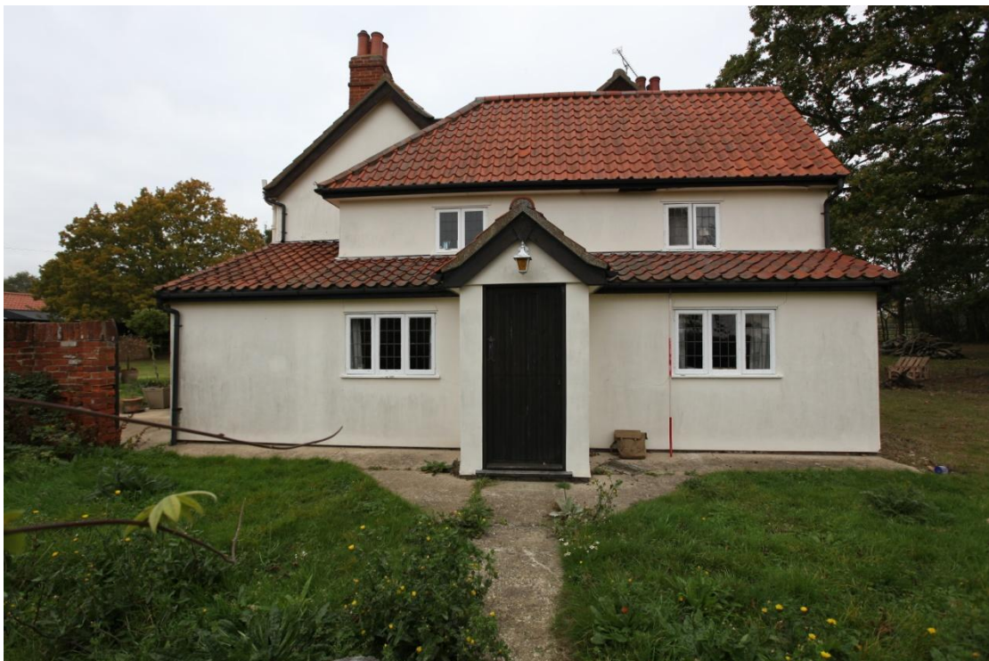
Illus. 2. The southern facade showing the hipped roof of the original 19th century structure (1) on the right behind its mid-20 th century lean-to extension (4). The north-western rear extension (3) is visible on the left.
