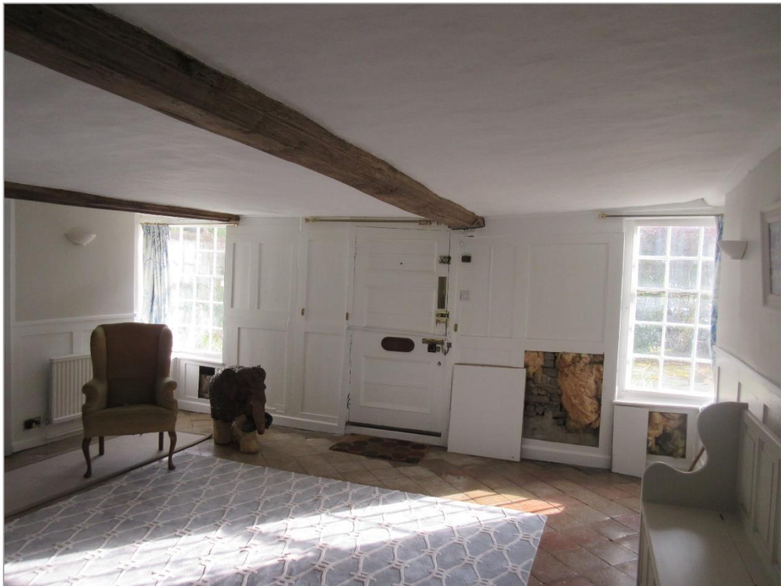
Figure 10: The entrance hall, view towards the front door, with the moulded and stop-chamfered spine beams of the late-C16 inserted floor and C17 and C18 panelling, some reset
