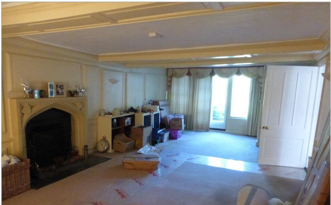
Figure 12: Drawing room, looking N. Previously two rooms, this was opened up to form a single space in the C20, with the panelling reused/replicated. The stone gothic fireplace is modern (Photo Rodney Black Design Studios)
