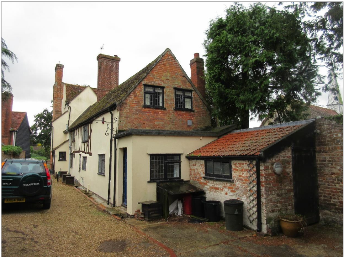
Figure 8: N range, looking S. This will be repaired and the negative/intrusive modern windows replaced with bespoke windows of more suitable design. The flat-roofed boot room will be given a pitched slate roof, and the brick shed slated and clad in shiplap boarding for insulation.
