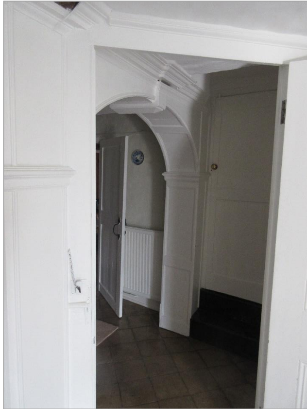
Figure 11: Removal of an inserted door and door frame (foreground) will allow the C17 arch to be returned to the entrance hall space
