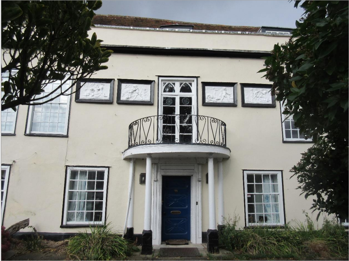
Figure 6: Front elevation. This will be repaired, with a new lime-based render finish. The inappropriate railings over the porch will be replaced with new railings of more sympathetic design
