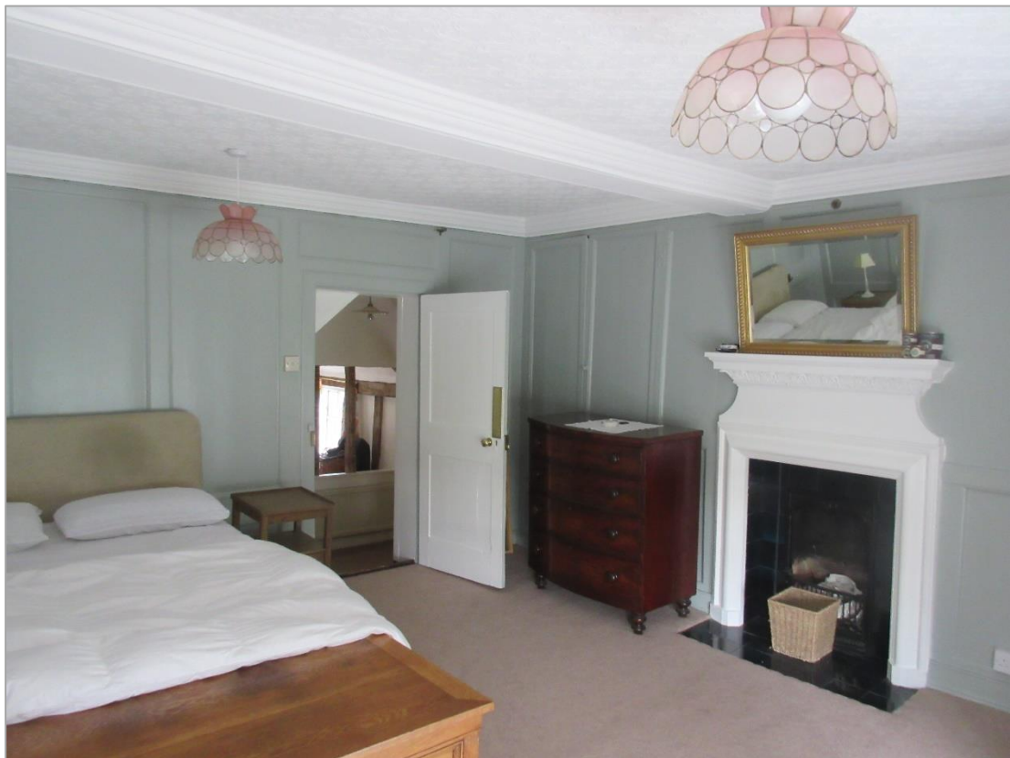
Figure 20: C18 raised and fielded panelling and chimneypiece in bedroom 2
