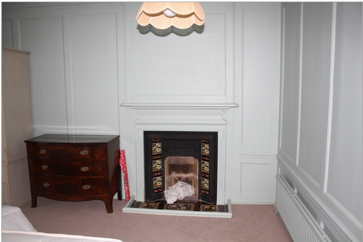
Figure 19: The western first floor bedroom will become the dressing room. It has C18 raised and fielded panelling and a C19 fireplace insert
