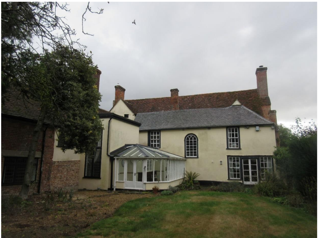
Figure 9: Rear elevation, with modern conservatory and flat-roofed stair addition to left. These will be removed to allow for the construction of the new stair turret and garden room. The modern French doors to the right will also be replaced.
