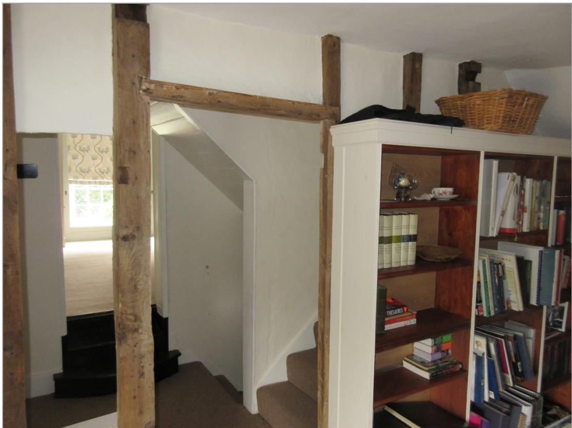
Figure 21: Inserted stud partition on first floor landing, looking south to bedroom 2
