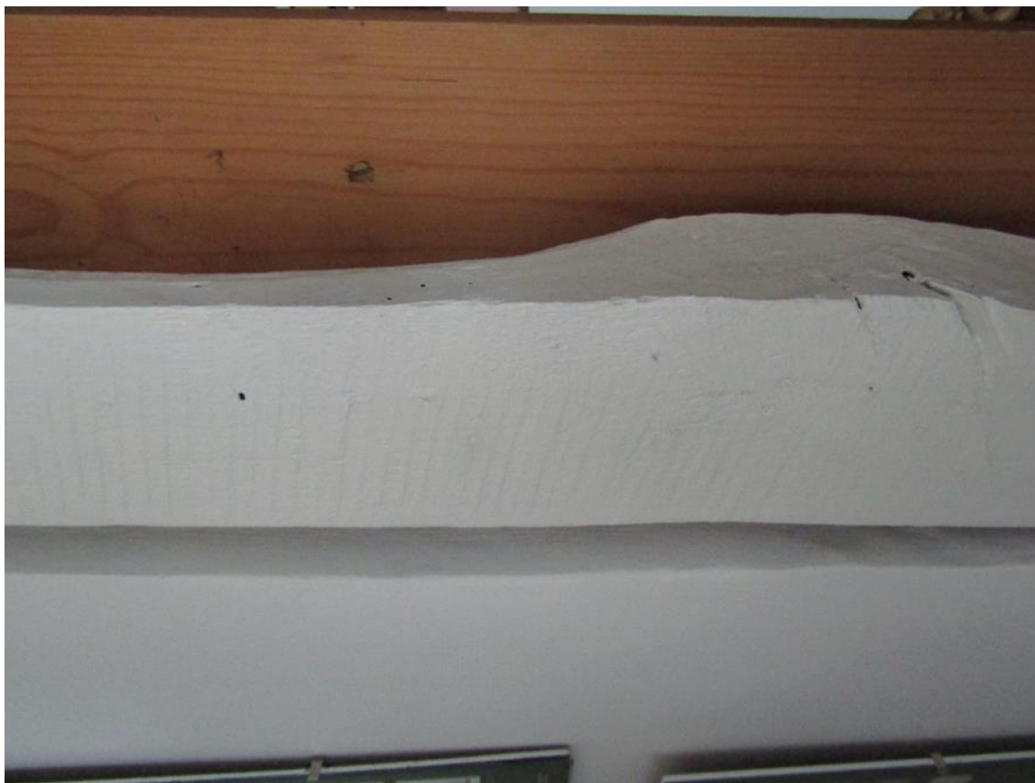
Figure 10 - marks of modern sawing on timber within Bedroom 3
