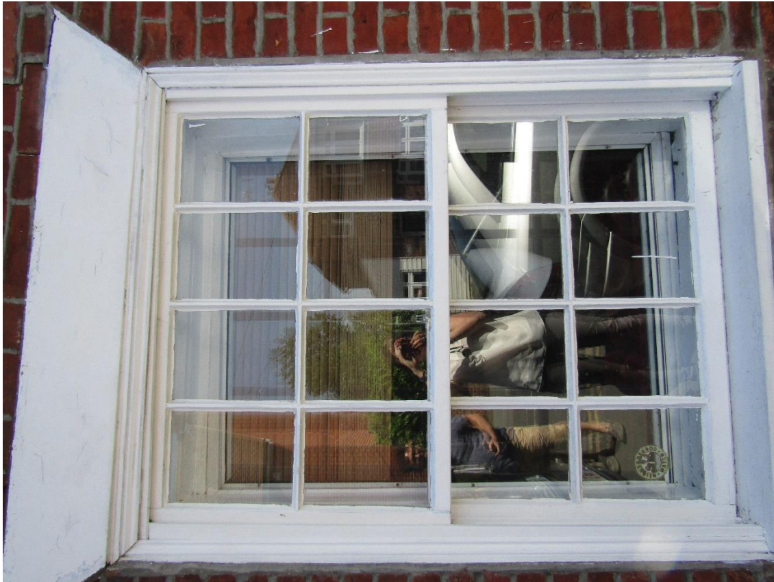
Figure 5 - ground floor sash window - reflection with secondary glazing
