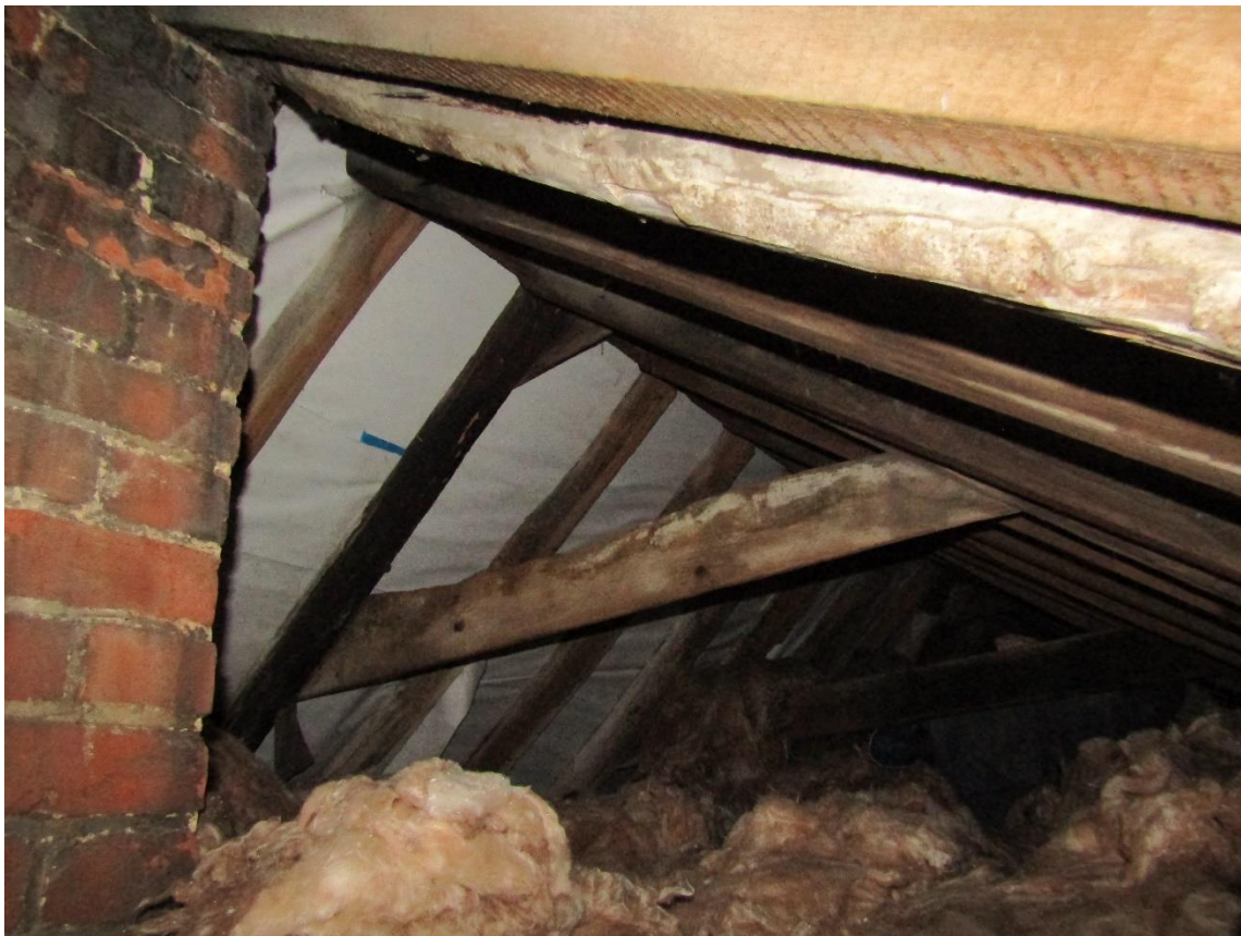
Figure 14 - historic water ingress on roof structure
