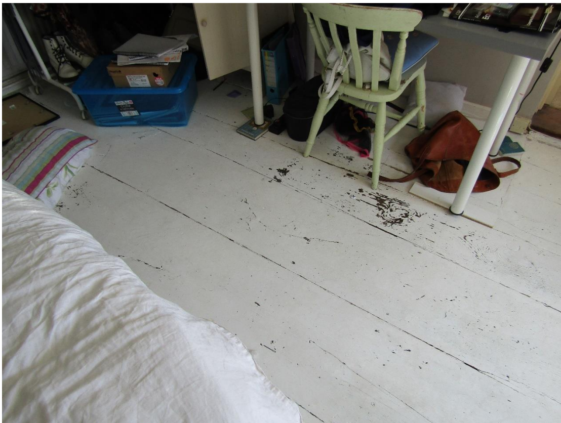
Figure 12 - wide floor boards indicating original floor boards
