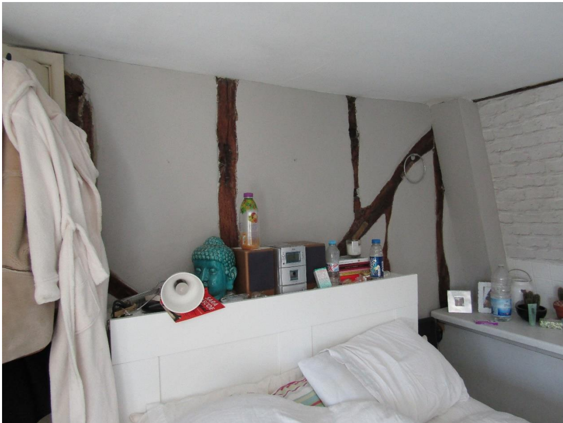
Figure 11 - exposed timber frame in Bedroom 2
