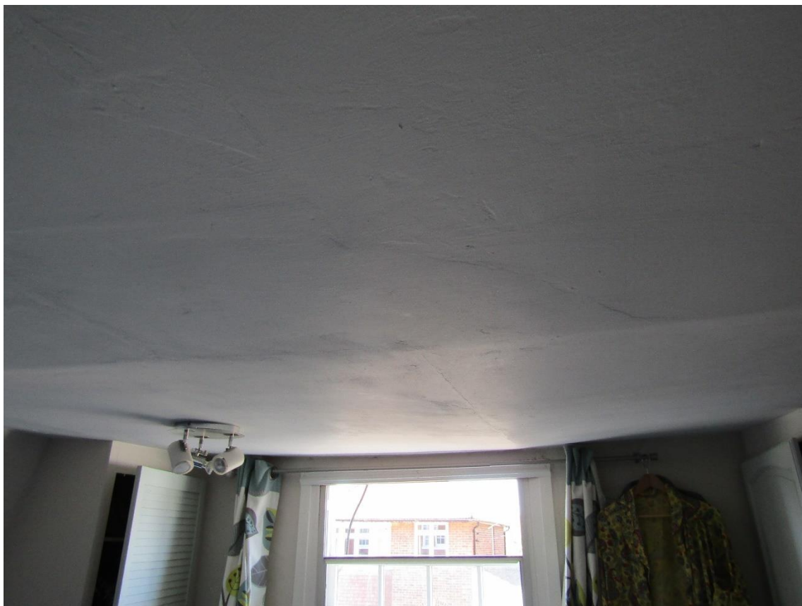
Figure 15 - ceiling in Bedroom 1 covered in Plaster board
