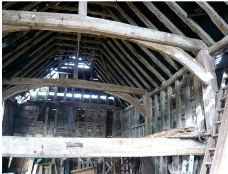
Plate 3: Interior of Grade 2*-listed barn showing crown-post roof
