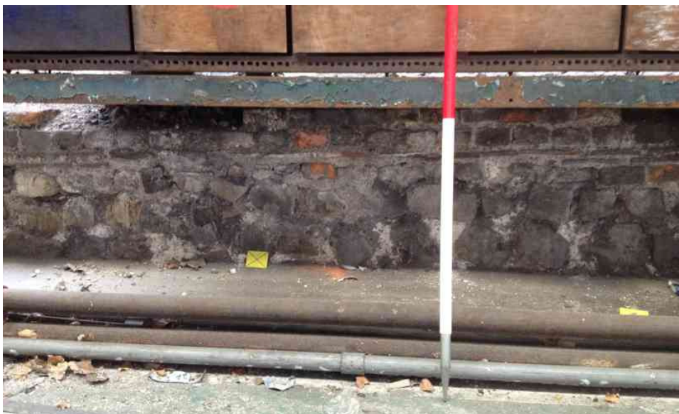
Plate 8: under lockers in Bay 2 the septaria is more regularly-coursed than elsewhere in depot, but this is not Roman-period.
