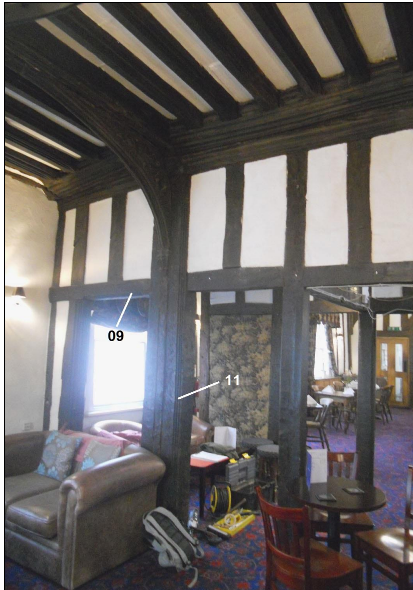
Figure 2: View of the east end of the cross-frame (from the north) between the ‘southern hall’ and the bar area (potentially Phase II), showing two of the timbers sampled (the other two from this frame being on the west side)
