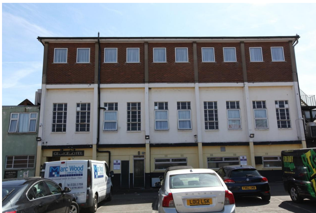
Illus. 5. The rear (northern) elevation from the car park on the site of the demolished stables. The painted ground and first storeys date from the 1930s, retaining their metal-framed Crittall windows, while the brick upper storey was added in 1984 or later. The green-painted structure to the left also dates from the 1930s. The ground floor originally housed the kitchens while the well-lit first floor was a dance hall (figure 9).
