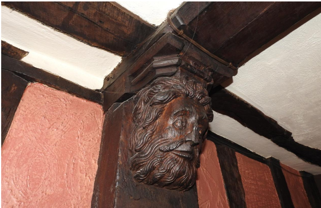
Illus. 25. The carved late-medieval or early-16 th century corbel block which is integral to the post supporting the main east-west ceiling beam of room 503 in the southern range (6f). In 1922 the Royal Commission wrote ‘On the ground floor the kitchen has a ceiling-beam with a curved brace resting on a corbel carved with a bearded head’. The kitchen may have been the area beneath the first-floor hall (2), which is likely to have been the principal room of the medieval inn. The ceiling of room 503 is a later insertion consisting almost entirely of re-used timber and appears to occupy the ‘gap’ of 1745. The incised patterns in its plaster are modern.
