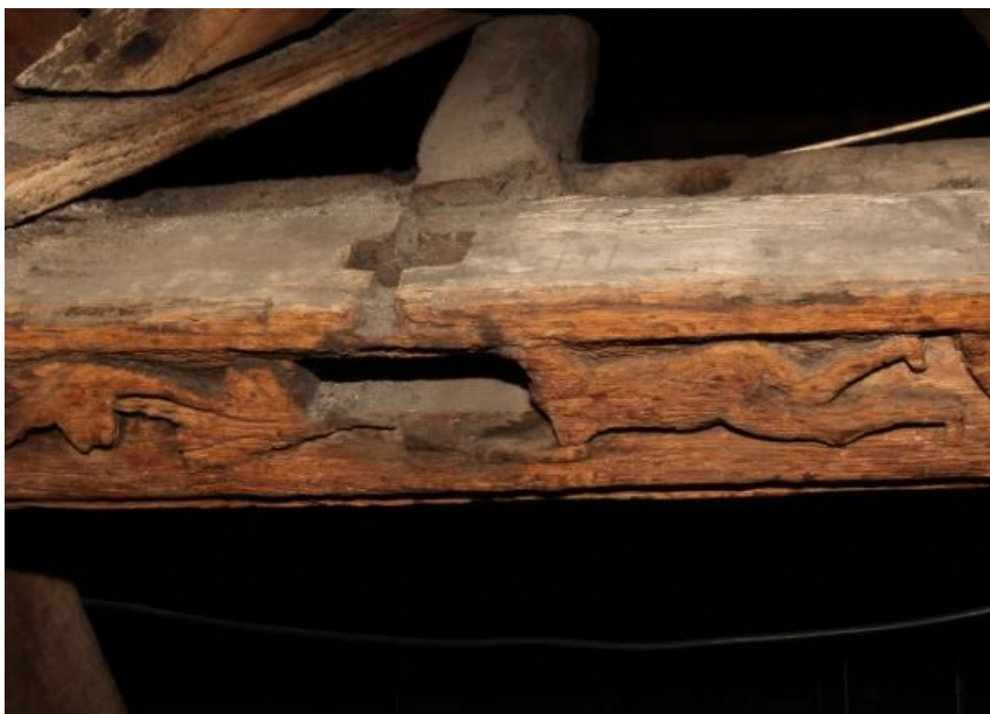
Illus. 32. A detail of a re-used carved mid-16 th century window sill in the 17 th century roof above room 305 (area 4f2). An apparently naked figure is holding a scroll of leaves. The roof contains many other re-used timbers, including sections of roll-moulded cornice similar to that of area 4 on the ground floor, but no others are carved.
