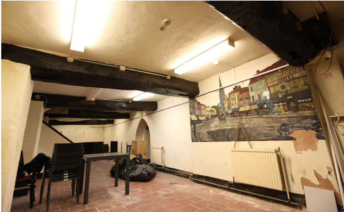
Illus. 10. The front (southern) section of the cellar viewed from the east, showing its massive 14 inch square ceiling joists with mortises for missing brackets at both ends. These brackets were presumably supported by missing corbel blocks in the walls. The 1922 Royal Commission describes two fireplaces with four-centred heads and ‘vent holes’ above their arches in the central spine wall on the right, along with a door beneath a two-centred brick arch that presumably equates to the present pointed doorway. The original wall fabric is now hidden by modern plaster and dry-lining.
