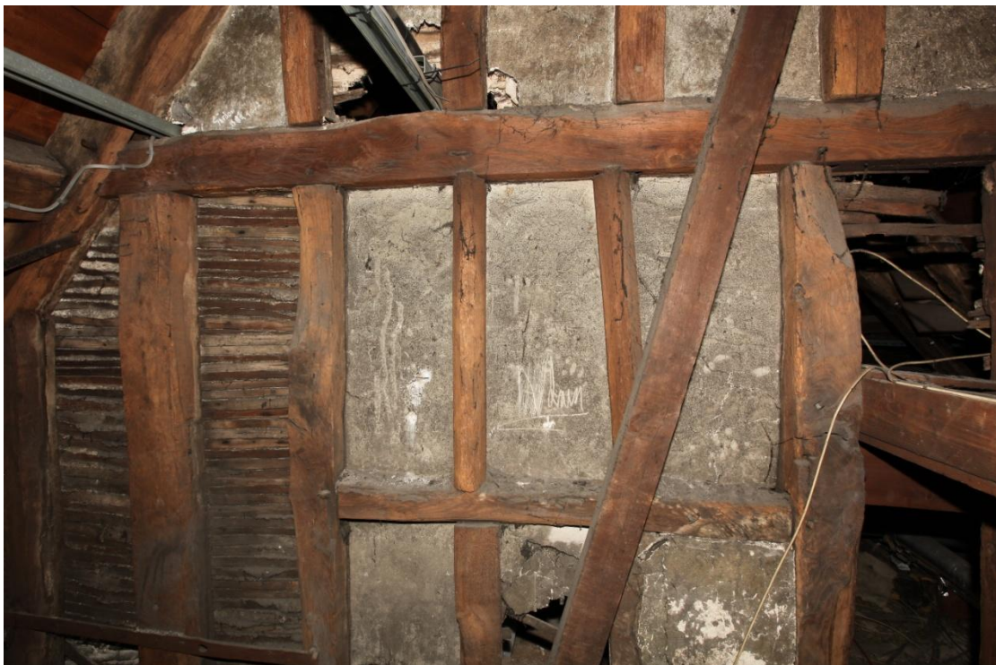
Illus. 29. A detail of the blocked 17 th century window with its two original chamfered mullions in situ . The tenoned mullions appear to be plainly chamfered externally as well.
