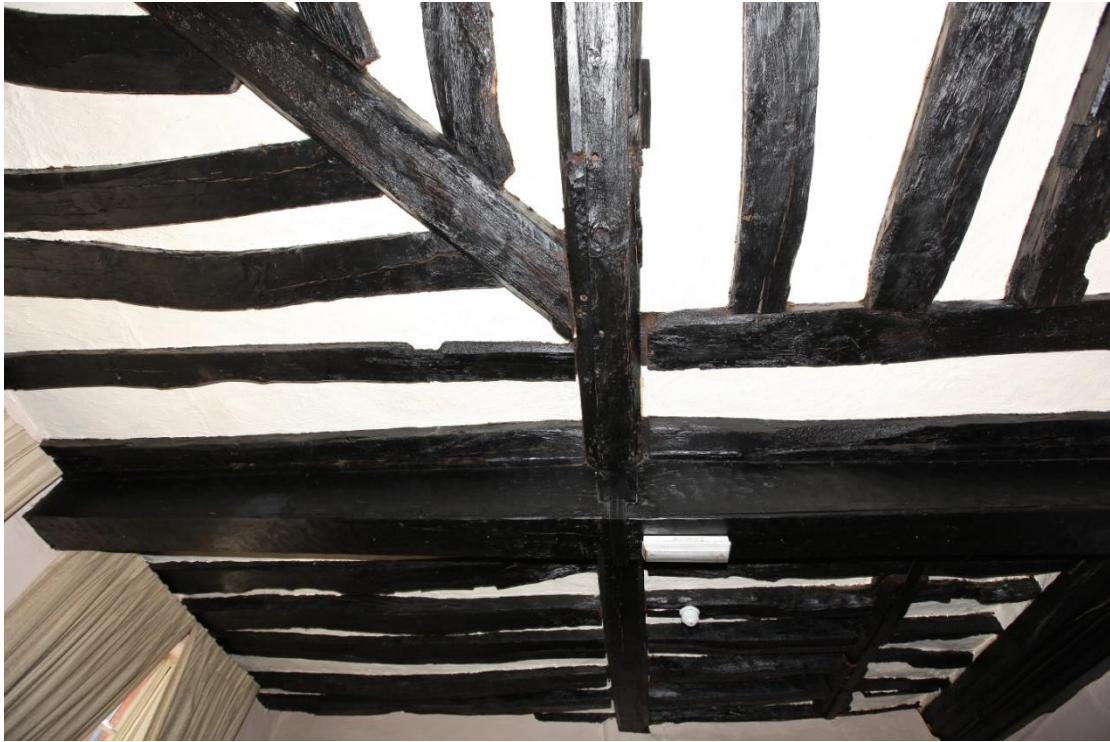
Illus. 14. The ceiling of the lounge on the corner of the High Street and George Street (4) viewed from the east. The central supporting beam is modern (possibly a boxed RSJ), but empty mortises for a missing original wall dividing the corner shop from another narrow room are visible immediately in front. A blocked trap is visible in the bottom right-hand corner for an original stair rising from the modern passage (illus. 15).
