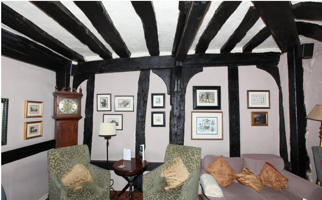
Illus. 13. The fine late-14 th or early-15 th century shop front in the eastern wall of the corner lounge (4). The right hand section was an open arched window, now with a later central post, and the two vertical studs on the left are the jambs of a blocked door. The two left-hand corner brackets are modern copies of the originals on the right. The moulded rail on the left is a re-used timber similar to others in the roof and the front wall on the right was formerly jettied but has been pushed out into the High Street. The roughly hewn, square joists are typical of the Middle Ages and are rare survivors in Colchester.
