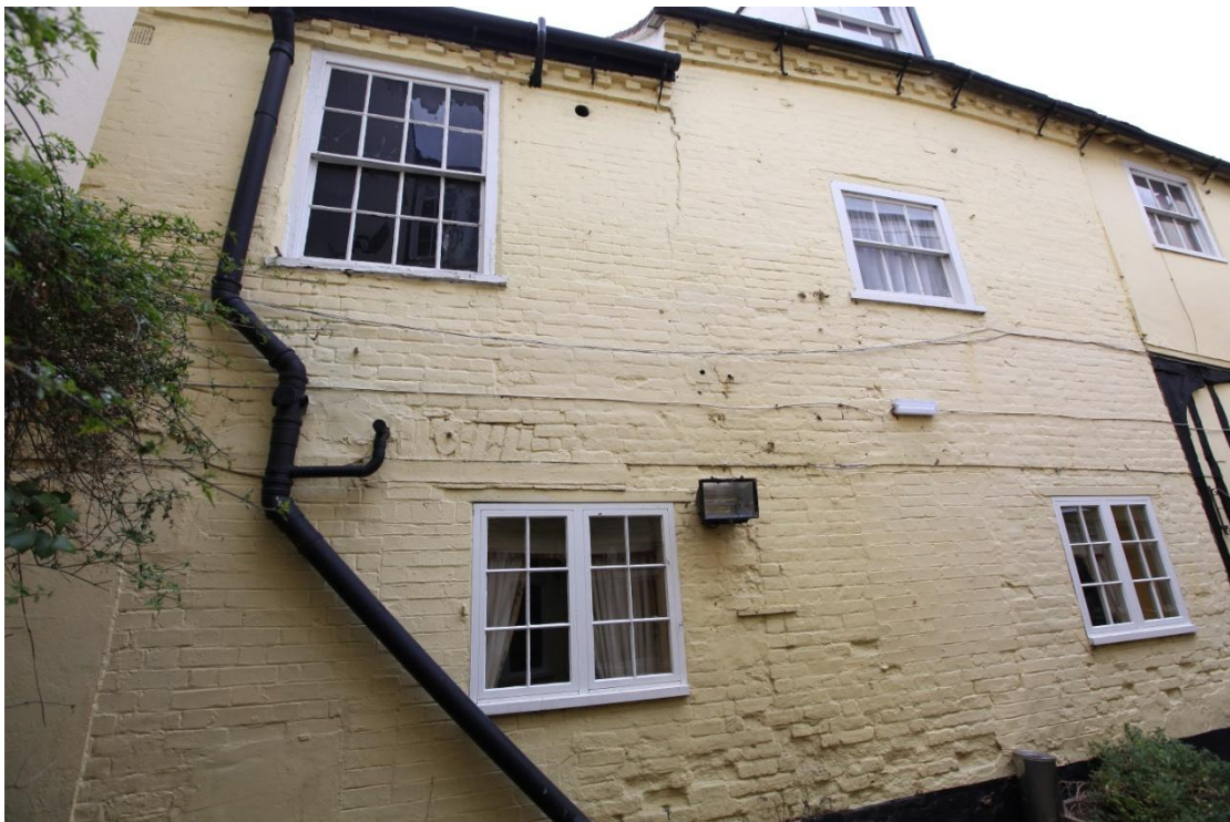
Illus. 9. The brick structure at the northern end of the courtyard's eastern range (9), with the gateway on the right. The brickwork is laid in Monk Bond (two stretchers between each header) and may date from as early as the late-17 th century, but has been much altered. A stable door opens into the ground storey in figure 13.
