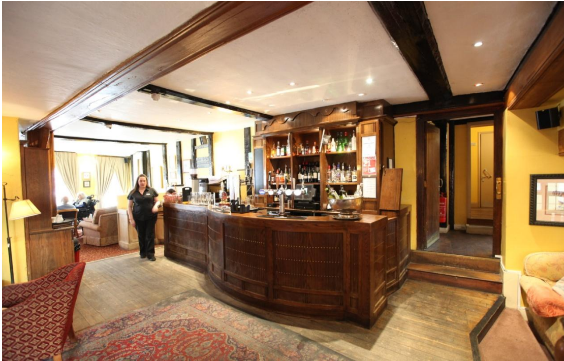
Illus. 18. The main bar seen from the east. This area (1) may have formed a medieval parlour, with a dividing wall beneath the brown-painted ceiling beam at top left, but has been much altered. The wall behind the bar adjoins the neighbouring early-16 th century structure at no. 117, but without further investigation of the fabric it is unclear whether its widely spaced studs are in situ or later insertions.
