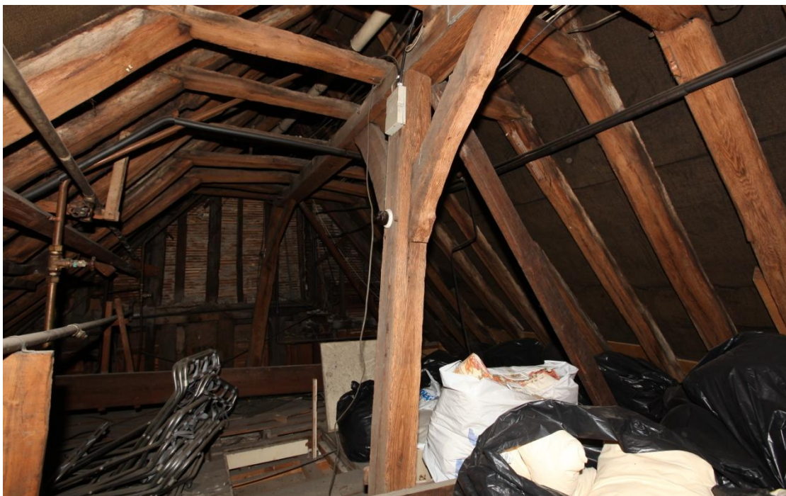
Illus. 27. The plain 15 th century crown-post in the southern section of the eastern range (7) showing the heavy studs and either the mid-rail or tie-beam of the earlier structure (3) in the rear (but not the roof-plate as studs survive both above and below).
