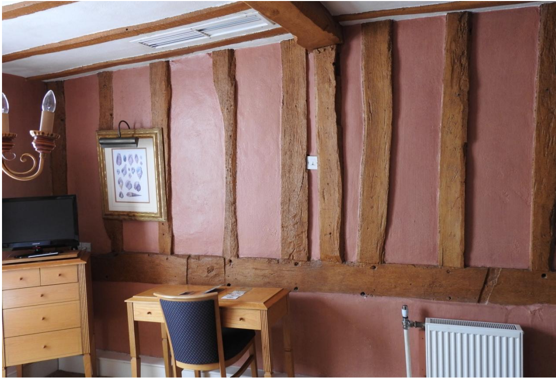
Illus. 26. The closely spaced early-16 th century studs of the eastern wall of room 307 on the upper storey – immediately above room 503 (6f2). This wall belongs to the adjoining high-status three-storeyed building at no. 117, and the room's inserted ceiling is supported by a later stud resting on its horizontal rail. The end of a jetty-plate is obscured by the chest of drawers to the right, and the roof gable above retains traces of external pargeting (illus. 31) so this room was formerly a gap in the street. The studs are not weathered and Roman carpenter's numerals are still visible at the foot of each.
