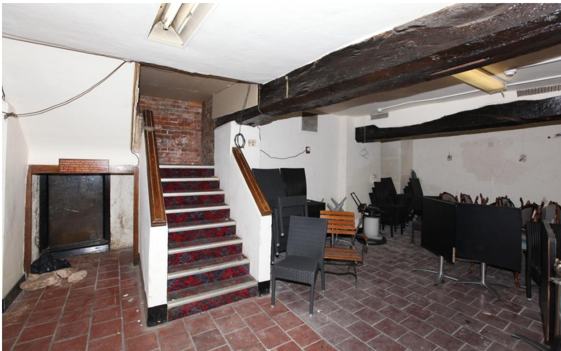
Illus. 11. The southern wall of the cellar showing the 20 th century staircase descending from the lounge above (area 5). This staircase is understood to have been blocked during the most recent refurbishment in the 1990s. The glazed niche in the original flint-rubble wall to the left exposes layers of archaeology which may include a Roman gravel pavement but not the reputed Boudiccan destruction layer.
