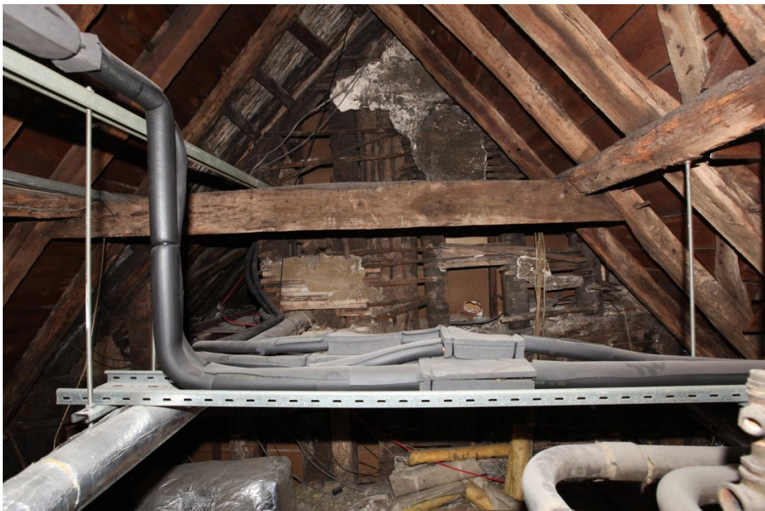
Illus. 31. The timber-framed wall of no. 117 from the roof above area 6. The plaster of this wall was also exposed to the street but is not decorated with pargeting. Instead it appears to be covered in a thick layer of brown paint – or dirt. The roof of no. 117 beyond is a later reconstruction visible in the attic room above no. 308.
