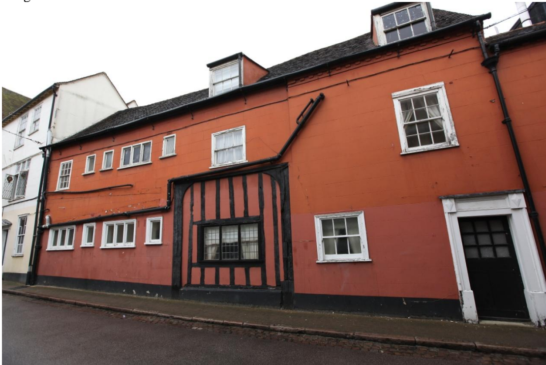
Illus. 3. The eastern range facing George Street, built in several stages. The section to the left of the gateway (7) is a 15 th century addition retaining its original crown-post roof (illus. 27), while the gateway – only blocked in the 1930s – is either contemporary or a slightly later addition with a rebuilt roof (8). Both structures have lost jetties and the gate posts contain mortises for foot-braces that projected into the street. The two structures of different heights to the right of the gate are of rendered brick, probably of the 18 th century but with 19 th century roofs (9 & 10).
