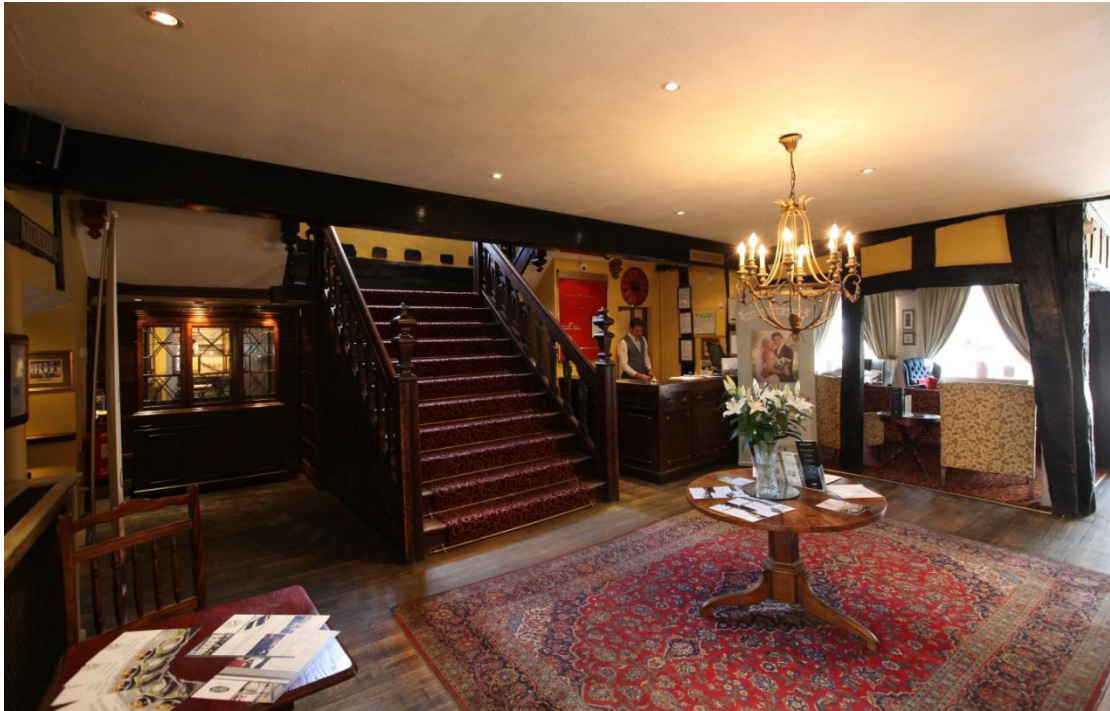
Illus. 16. The hotel's reception area (3) showing the Victorian Mock Gothic staircase on the left and the entrance passage on the extreme right. This area formed part of the medieval structure and must have been sub-divided, but has been much altered and concealed. The cut-off ends of the jettied ceiling joists adjoining George Street are visible above the staircase, and both posts on the right appear to be later insertions.
