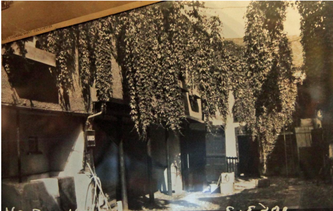
Figure 14. The overgrown open-sided elevation of the western courtyard range before the construction of the present bay-fronted single storied extension between 1933 and 1943. There is no trace of the upper storey with its gallery and continuous windows which was presumably added at the same time. From a photograph on display in the hotel's reception (with an overlapping postcard obscuring its top left-hand corner).
