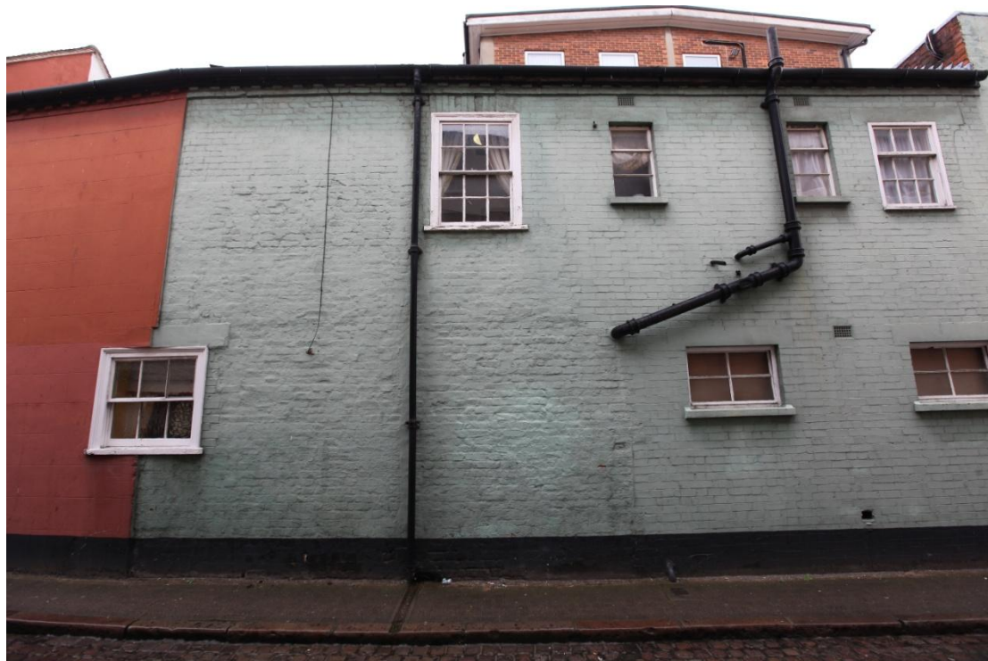
Illus. 4. The George Street frontage showing the junction between the worn 18 th century brickwork in Monk Bond (9 & 10) and the new work of the 1930s (i.e. between 1933 and 1943) to the right of the diagonal pipe. The upper courses of the 18 th century brickwork were renewed in the 19 th century. The 1980s addition is visible above (14).
