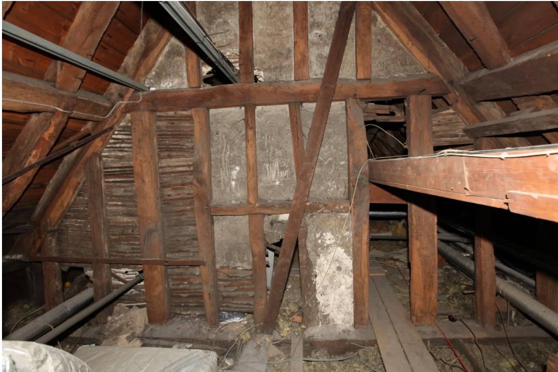
Illus. 28. The blocked window in the internal western gable of the 17 th century roof above the High Street range (i.e. above area 5 on the ground floor, looking east to area 6). The roof structure of staggered butt-purlins consists largely of re-used timber, with the rafters interrupted by the purlins. The feet of the rafters have been truncated by the present High Street wall on the left and originally projected by approximately 18 inches further – forming a jettied second storey. The boarded channel on the right contains modern pipes.
