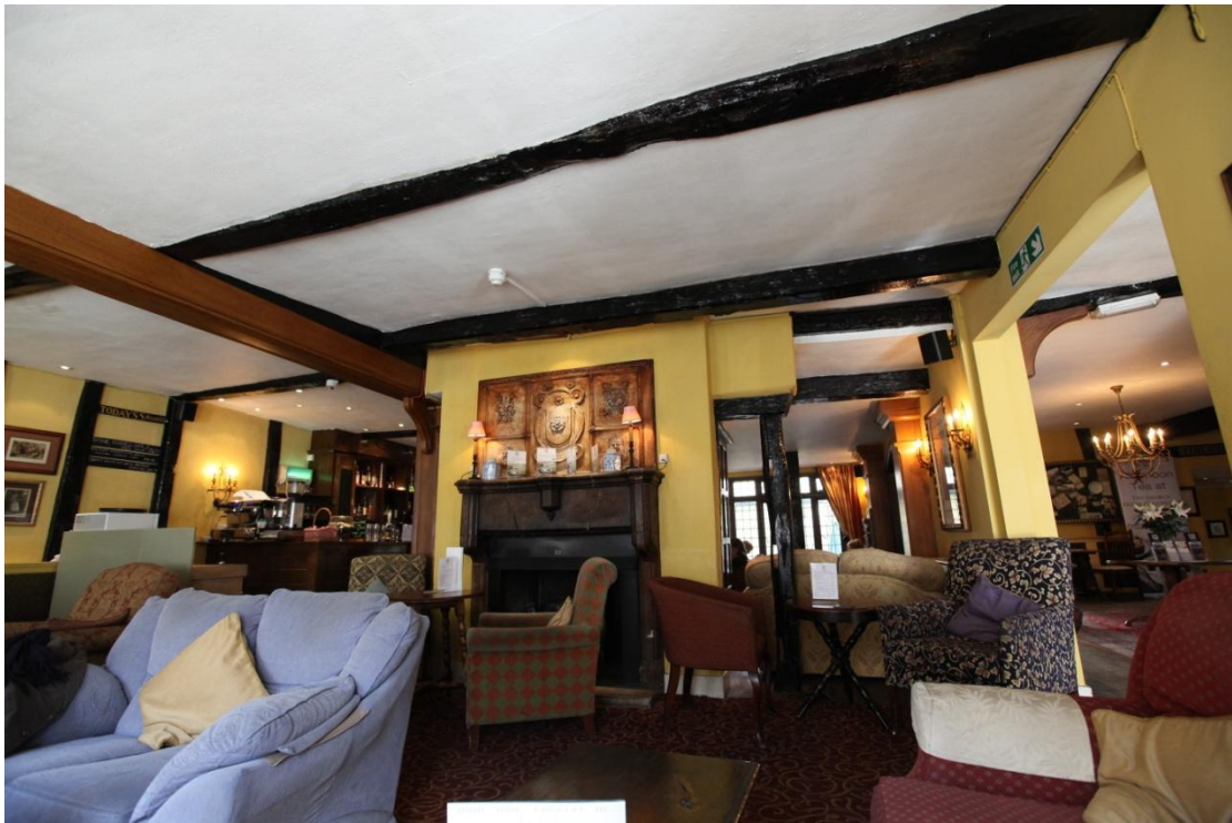
Illus. 17. The front lounge showing the central 15 th century-style fireplace resting on the spine wall of the cellar. Whether this chimney contains any early fabric is unclear. This area (5) lies beneath the 17 th century roof with a window above the brown-painted ceiling beam on the left, and the area occupied by the bar (6) beyond was an open passage linking the High Street to the rear yard as shown in 1745 (figure 3).
