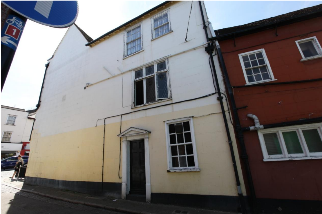
Illus. 2. The eastern elevation to George Street with an original Georgian triangular door pediment. The white area appears to have part of the original late 14 th century building with the shop front shown in illus. 13 to the left. Its jettied (overhanging) first storey has been cut off, as has the jettied second storey of its 17 th century upward extension. The roof timbers of the present roof gable at top left have been truncated.
