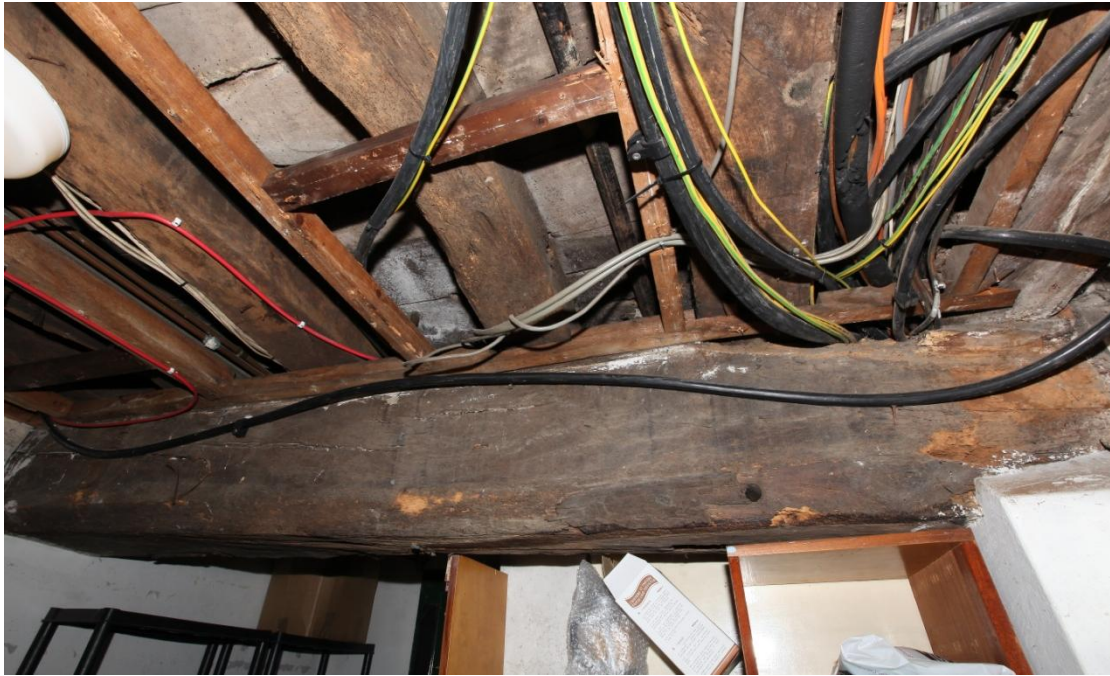
Illus. 12. A detail of the ceiling in the rear (northern) half of the cellar, viewed from the east (in the maintenance workshop). The common joists are lodged on top of the principal joist rather than tenoned to it, in a manner usually found only in the 13 th century or before. Some of the rear principals contain bracket mortises but others don't.
