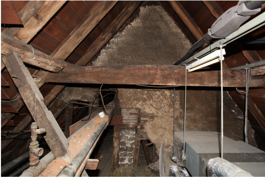
Illus. 30. The exterior of the gable shown in illus. 28, looking east from the later clasped-purlin roof above area 6 on the ground floor, with the blocked window in the centre. The lime plaster is decorated with a basket-weave pattern which pre-dates the blocking of the window and was clearly exposed to the street as indicated in 1745 (figure 3).
