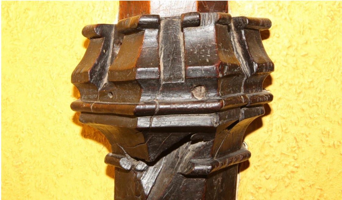
Illus. 24. A detail of the carved crenellated capital of the crown post. This is a fine piece of medieval carving which may be contemporary with the late-14 th century hall but is also consistent with a 15 th century date. It is not in situ and there is no guarantee it was not re-used from elsewhere like many other timbers in the inn.
