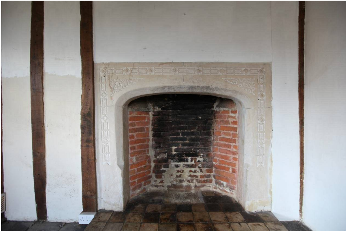
Illus. 10. The fine original stone fireplace in the parlour chamber (i.e. the bedroom above the drawing room as labelled in figure 7). Many early-17 th century fireplaces used plaster to imitate stone, but this is entirely genuine and represents a rare survival. The brickwork retains original red-ochre pigment, and the whitewash above may conceal a contemporary overmantel painting.
