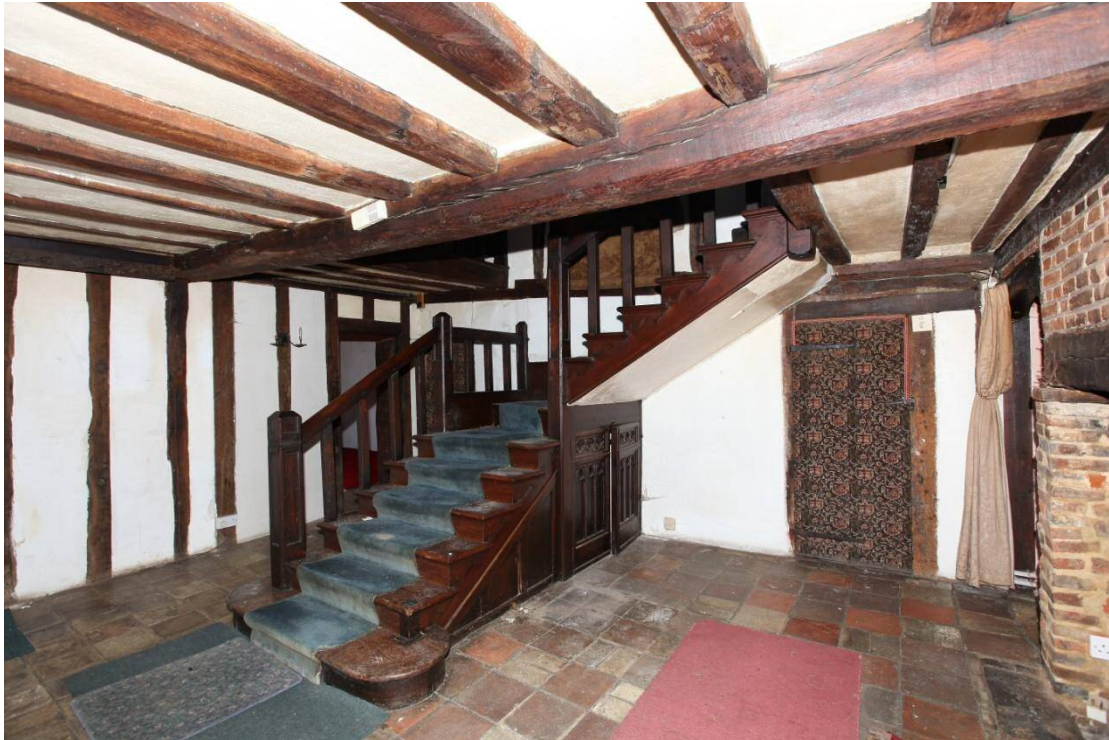
Illus. 8. The rear hall (reception hall) from the east, showing the solid Arts and Crafts style 1930s staircase from which the right-hand hand rail has been removed.
