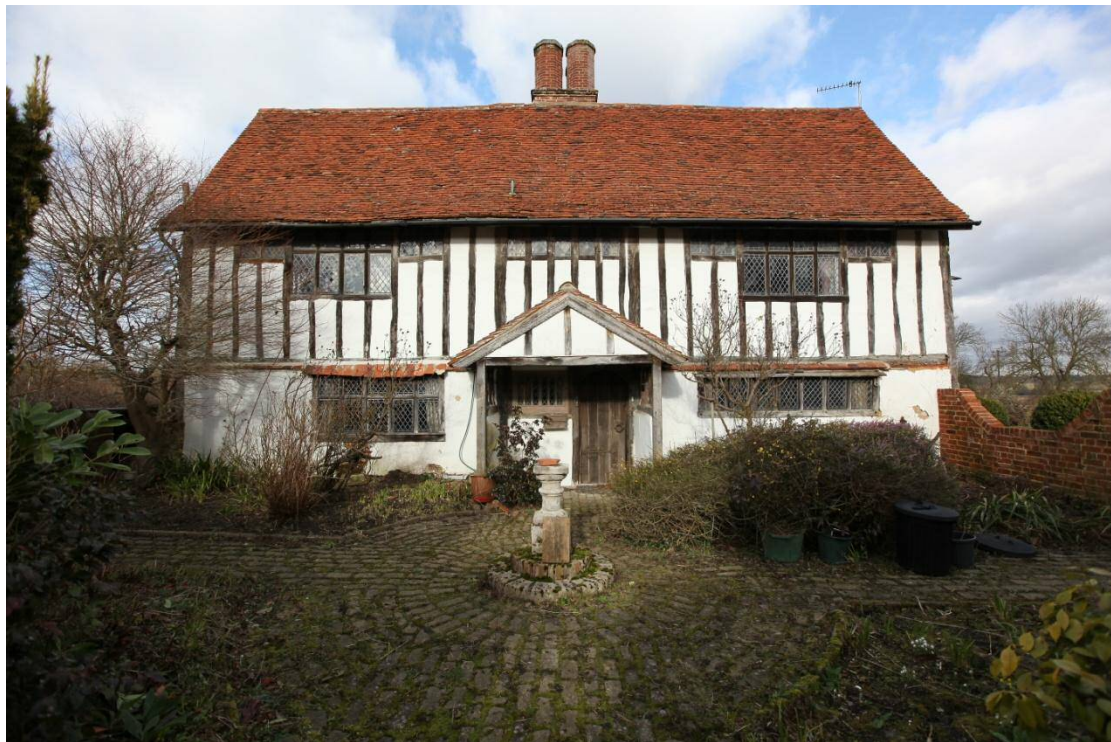
Illus. 1. The southern facade, showing the 1930s porch in the centre. The roof-plate contains mortises for an original two-storied porch and there is evidence of a blocked first-floor door immediately above the present entrance. The side-lights of the main first-floor windows contain 17 th century ovolo-moulded mullions, but the glazing and other mullions date only from the restoration. The original principal windows projected from the facade, and the timber frame was rendered and probably pargeted from the outset.
