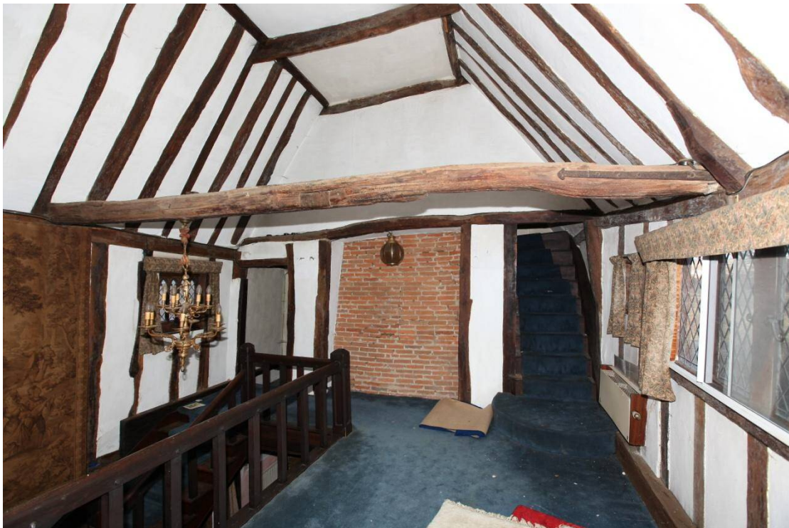
Illus. 13. The chamber over the rear hall (reception hall) from the south. Many timbers in this section of the house are soot encrusted but contain mortises that bear no relationship to their present positions and were re-used in the 17 th century from a medieval open hall that may have occupied the same site.
