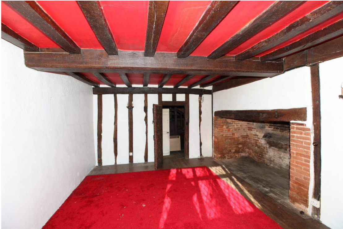
Illus. 6. The main hall (dining room) from the south. The studs of the rear wall have been altered, and the position of any original door is unclear, but the large fireplace to the right is largely intact beneath its original ovolo-moulded (quarter-round) timber lintel. The internal brick partition on the left is a relatively modern insertion of the late-19 th century or possibly the 1930s (indicated by a dotted line in figure 6).
