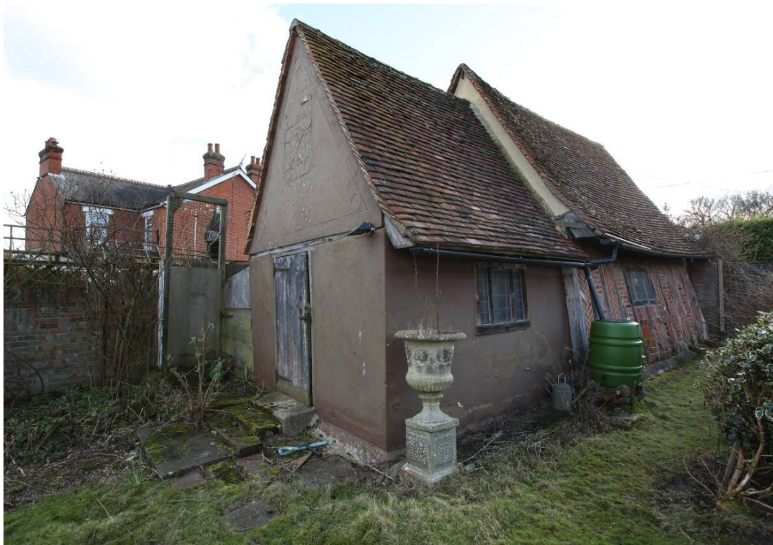
Illus. 15. The outbuilding adjoining the eastern boundary of the garden, viewed from the north-west. The taller section to the right, with a brick-infilled frame of re-used timbers, dates from the 1930s restoration, but the section in the foreground is a later extension. Both have been re-roofed in recent years and are leaning perilously.
