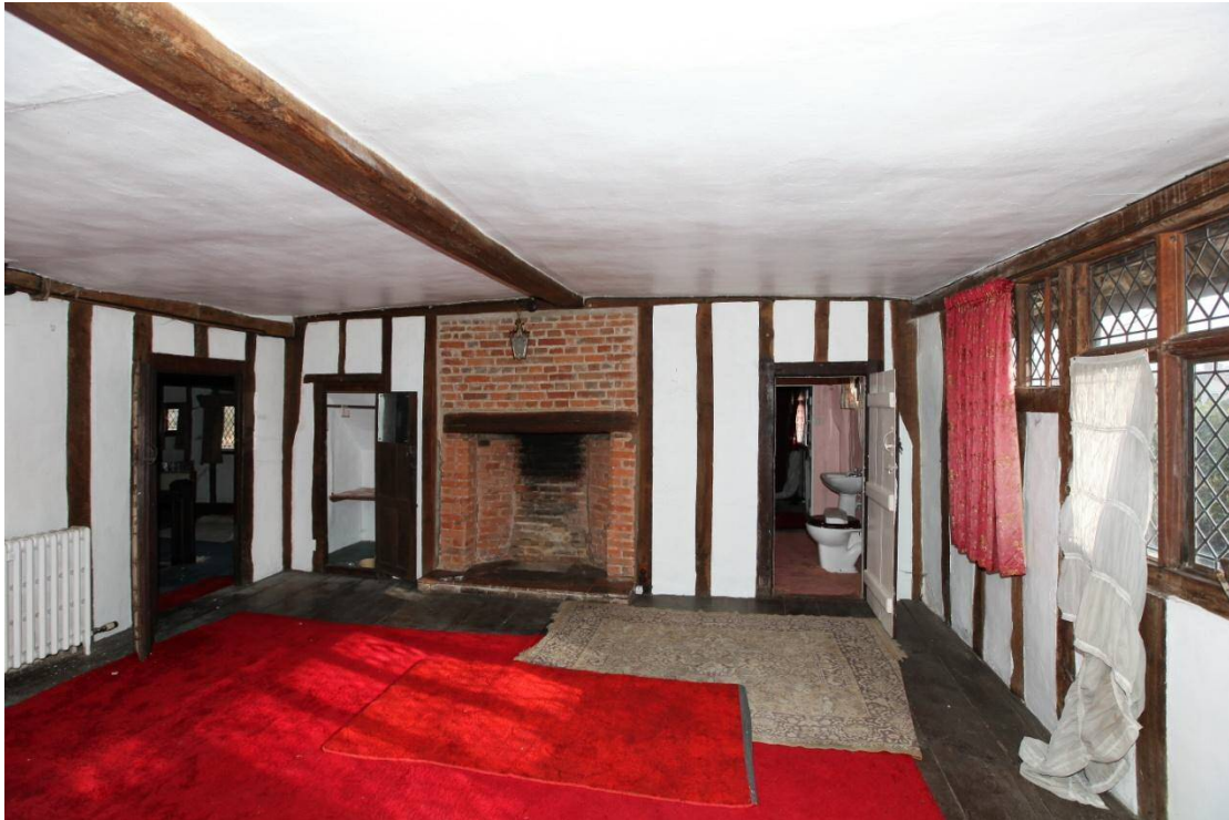
Illus. 12. The hall chamber (the bedroom over the modern dining room) from the west. The fireplace is original, with an ovolo-moulded lintel and red-ochre to the brick piers, but the upper brickwork would have been rendered. The door on the right would have given access to the original stair landing, and to the small chamber above the two-storied porch.
