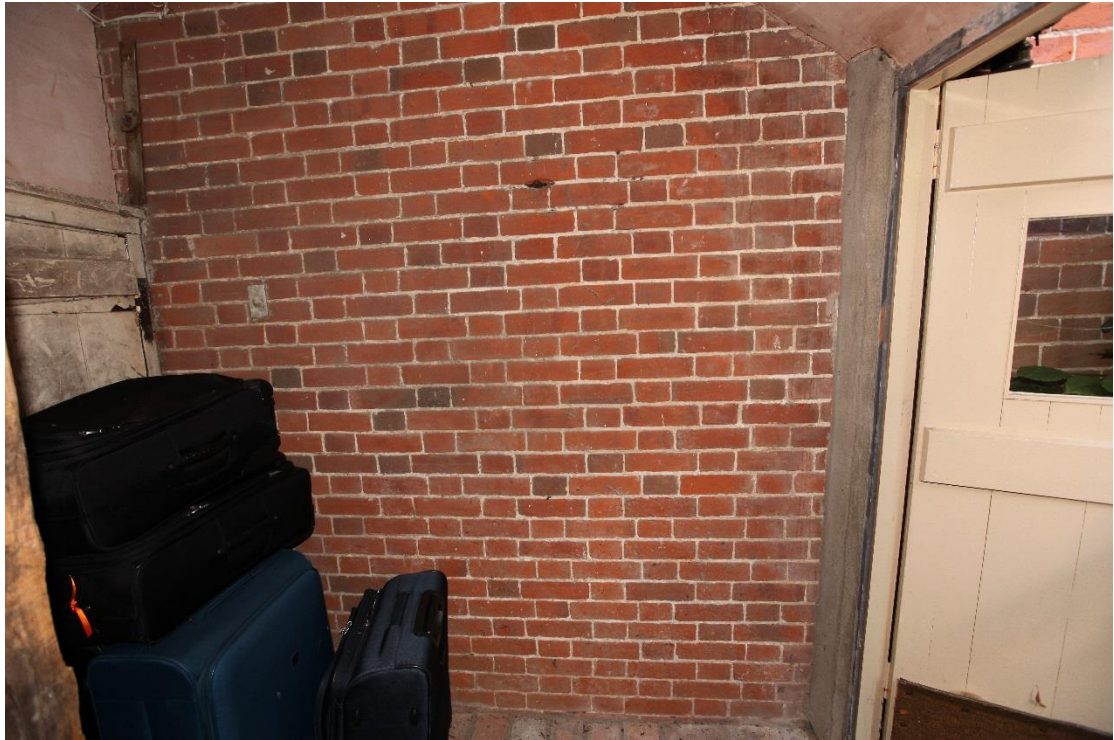
Illus. 11. The southern external wall of the brew-house seen from the secondary ‘lobby’ (figure 9) which now links the structure to the main house - the corner post of which is visible to the left. It should be possible to insert a new door to the right of this wall and so avoid damaging the internal pump in the south-western corner of the brew-house.
