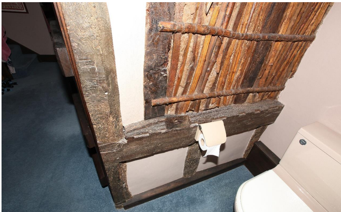
Illus. 6. The intact central section of the tie-beam which spanned the width of the 16 th century open hall, seen from the east. The pegged mortise in the centre of the beam (to the left of the toilet-roll holder) held a crown-post which supported the original roof, but this was rebuilt in the 17 th century when the present wattle-and-daub partition was inserted. The left-hand section of the beam is interrupted by a 17 th century door frame.
