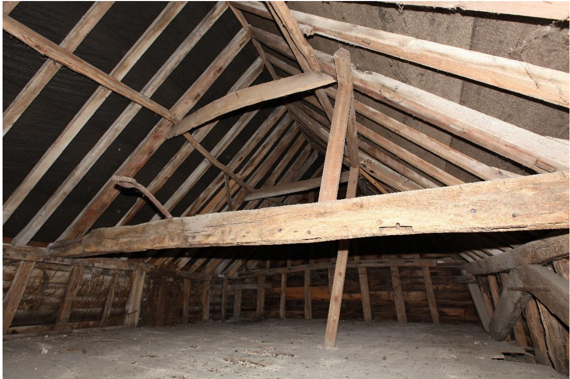
Illus. 15. The loft above the timber-framed stable (B), seen from the north. Almost all the timbers visible here have been re-used from one or more older structures in a manner typical of the 18 th century. The (re-used) rear roof-plate to the left contains an edge-halved and bridled scarf joint of the 16 th century.
