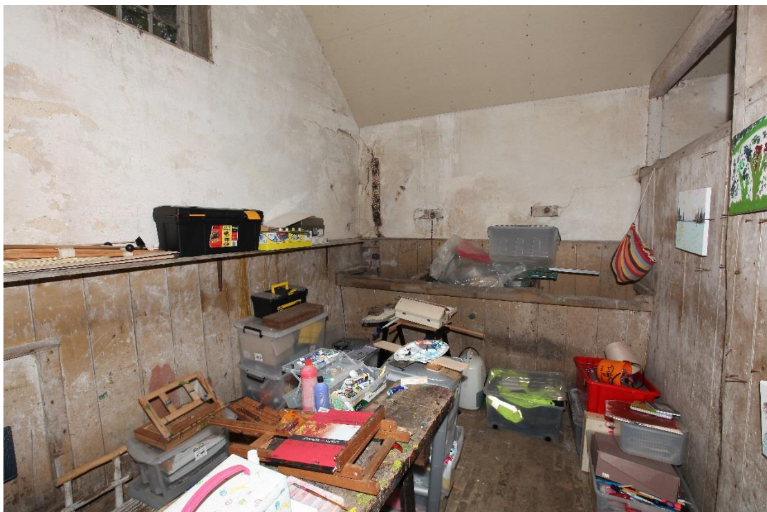
Illus. 18. The stall with its original boarded manger at the northern end of the 19 th century red-brick stable, viewed from the west. The wainscot consists of narrow painted boards in contrast to the much larger horizontal boards of the 18 th century stall to the south. A small aperture in the northern gable to the extreme left was designed to assist mucking out and is a common feature of early stables.
