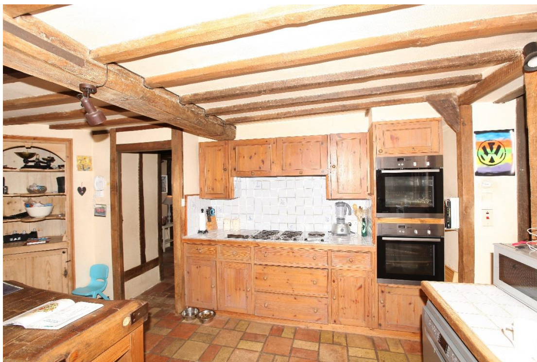
Illus. 4. The kitchen from the east (as named in figure 9) showing the intact 17 th century ceiling which interrupts an earlier arch-brace in the top right-hand corner. This brace rose to the tie-beam of a barn-like open hall before the ceiling's insertion.
