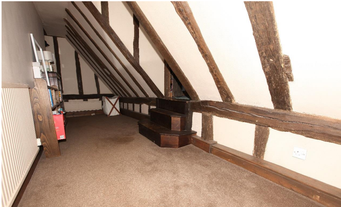
Illus. 5. The first floor corridor immediately above the kitchen, seen from the east. The roof-plate to the right of the steps (which lead to the upper chamber of the ‘closet’ tower) contains a dovetail joint for the missing horizontal tie-beam to which the bracket in illus. 4 originally rose. The central section of the tie-beam survives intact beyond the 20 th century partition to the left (illus. 6).
