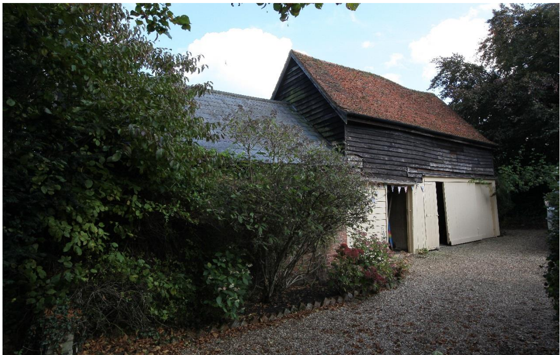
Illus. 12. The western façade of the stable from the north-west. The single-storied red-brick structure on the left is a well preserved mid-19 th century stable with its original fixtures and fittings (area A in figure 8). Two windows are hidden behind the undergrowth. The timber-framed structure was probably built as a stable, cart shed and hay loft in the late-18 th century (B); the sliding doors to the right-hand section are insertions of the 20 th century but much of the chamfered weatherboarding is original.
