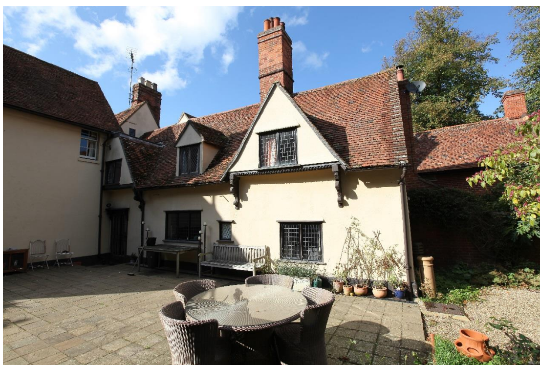
Illus. 3. The best preserved section of the southern façade to the east of the Victorian extension which retains fine early-17 th century brackets beneath its projecting gables. The brew-house is visible to the right.
