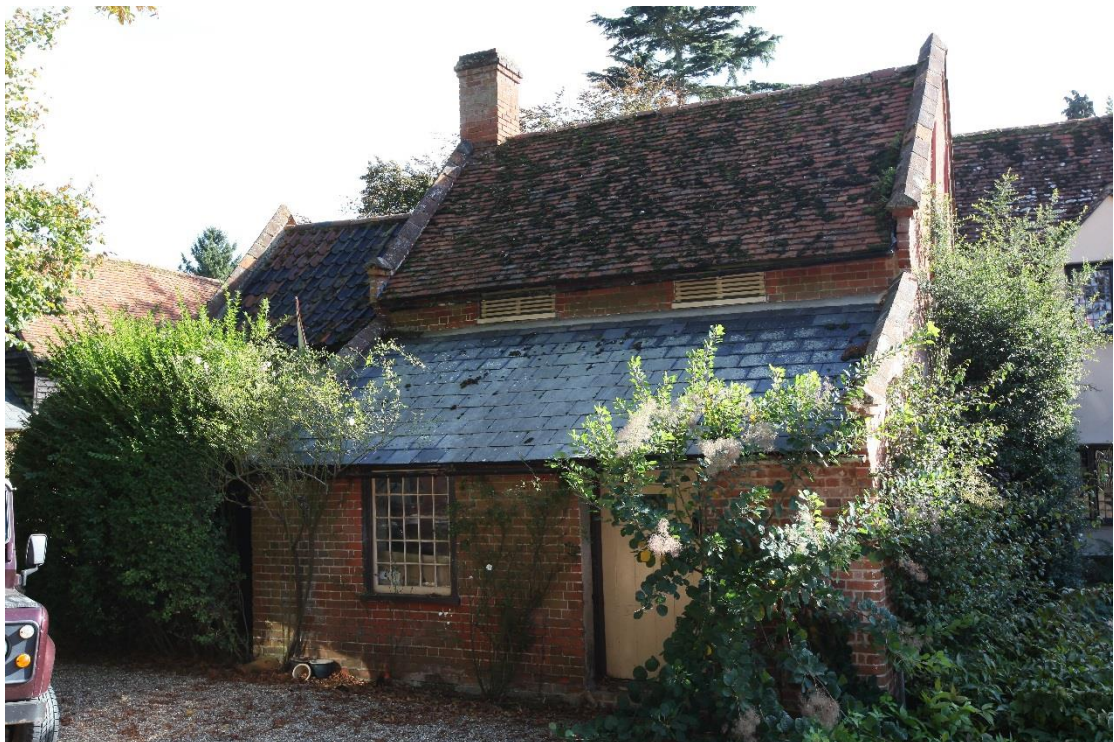
Illus. 8. The unusually well-preserved red-brick brew-house seen from the north. Despite their different roofs the slate lean-to in the foreground and the pantiled shed on the left are integral to the peg-tiled structure. Note the original ventilation louvers above the lean-to wood store. The right-hand (north-western) corner of the lean-to has been rebuilt and its present doorway occupies the position of an original window.
