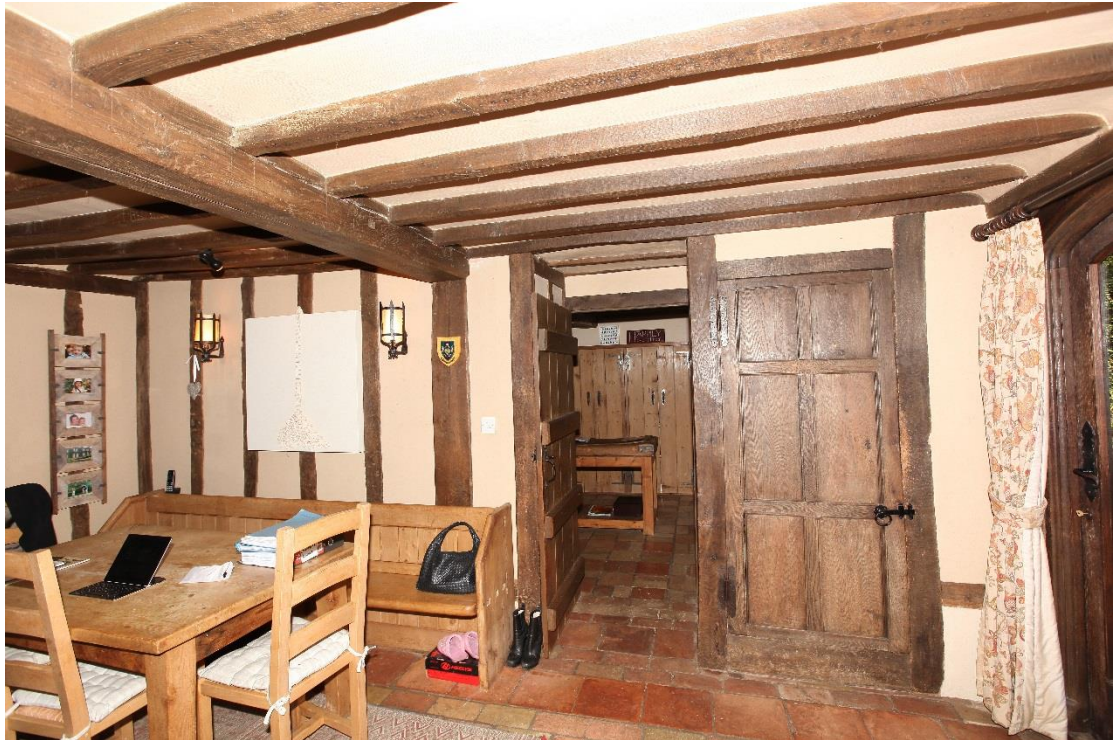
Illus. 7. The dining room from the west, showing the entrance to the kitchen. The dividing partition consists of old timbers and incorporates a 17 th century panelled door, but is a 20 th century insertion that post-dates the removal of lath-and-plaster from the ceiling joists. The dining room and kitchen originally formed a single hall.
