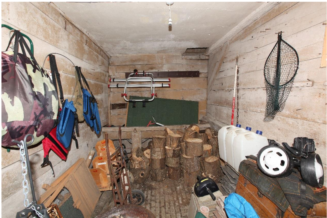
Illus. 16. The stall at the northern end of the timber-framed stable, which retains its impressive late-18 th century boarding and brick floor along with a mid-19 th century wooden manger. The diagonal scar of a missing hay rack can be seen above the manger to the right. John Constable may well have used this very stall on his visits to the house.
