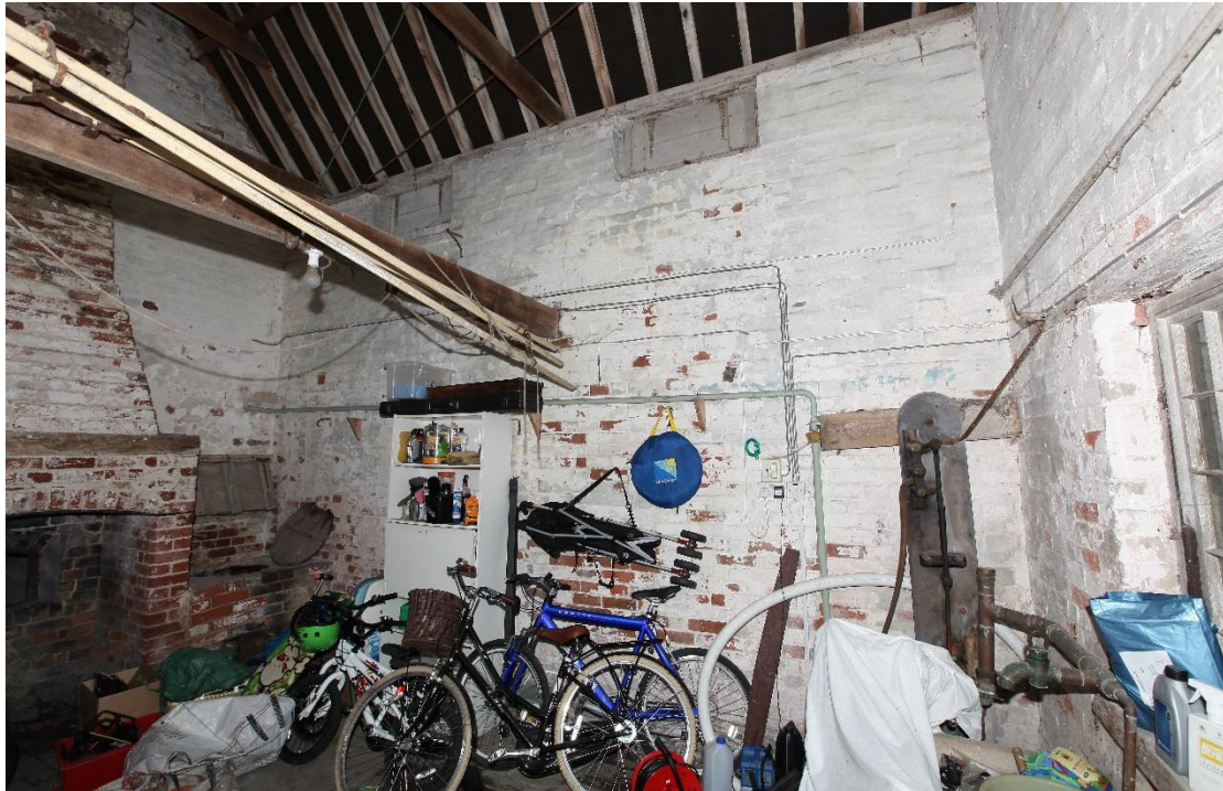
Illus. 9. The southern interior of the brew-house with pump and sink to the right and chimney to the left. Note the vertically hinged shutters to the ventilation louvers matching those of the opposite wall shown in illus. 8. The space has never contained a ceiling and the wooden beam spanning the walls retains a number of meat hooks.
