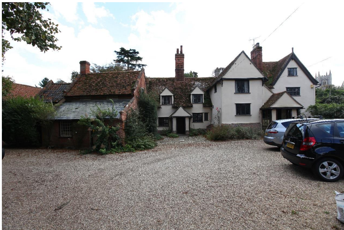
Illus. 1. Mill House from the north, showing St Mary's church to the right, the red-brick brew-house to the left and the roof of the stable to the extreme left. The low section of the house in the centre was built as an open hall in the 16 th century and the right-hand parlour cross-wing was added in the 17 th century. The central wing is also a 17 th century addition and appears to have formed a rare 'closet' tower with an integral cellar.
