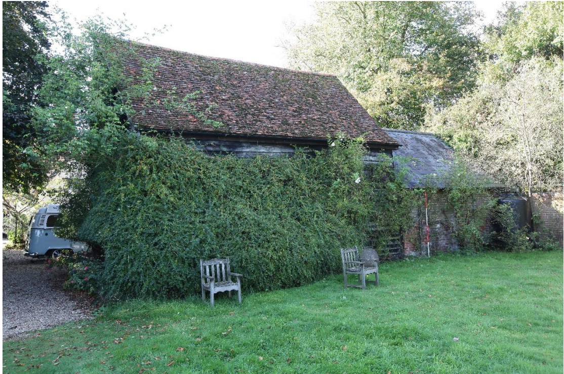
Illus. 13. The stable range from the rear (east). This elevation lacks windows and doors as in the typical manner of early stables which contained mangers and hay racks against their back walls. The tarred weatherboarding of the timber-framed section to the left appears to be intact behind the vegetation.
