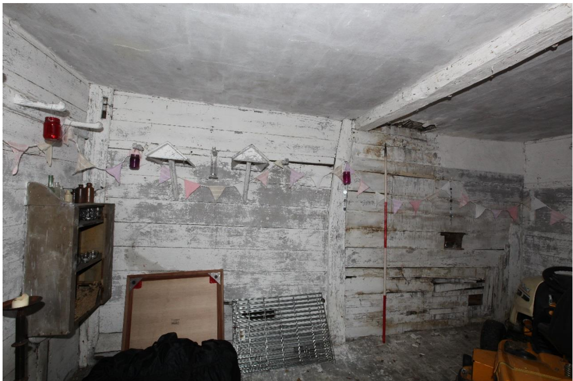
Illus. 14. The rear (eastern) internal elevation of the southern section of the stable, now used as a vehicle shed but with 19 th century wooden harness hooks visible to the left. The walls consist chiefly of re-used 16 th or 17 th century timber but it is possible that a small section survives in situ behind the ostensibly original boarding at lower levels.
