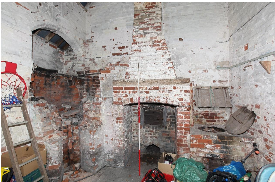
Illus. 10. The impressive original bread oven at the eastern end of the brew-house, with a slightly later copper to the right. The vertically hinged shutter above the lidded copper conceals a series of ventilation loops in the brickwork. The domed oven is intact behind its iron door with an ash hole beneath. The partly destroyed brick structure to the left probably supported a large brewing copper approximately 1 m above the floor, but this has been removed.
